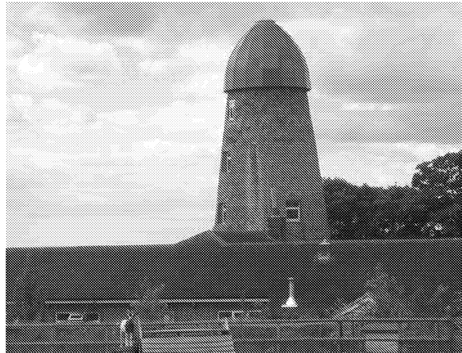
Figure 7: Ecclesden Mill, within the parish of Angmering. Built in 1826, the mill was originally called Highdown New Mill. In 1872 milling ceased and eight years later, the sails were blown off in a storm. Today, the mill is a private residence and has recently been heightened and had a new lead cap added (S. Carey).
