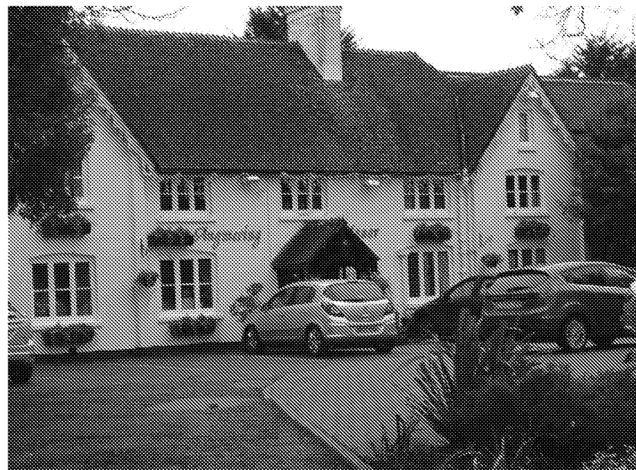
Figure 8: Angmering Manor. Originally the Rectory, this building is a mixture of 17th and 19th century construction.
