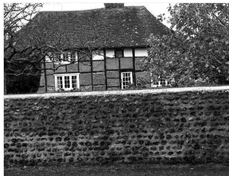
Figure 37: This approx. seventeenth century timber-framed house with red brick infill, sits to the south of the High Street.
