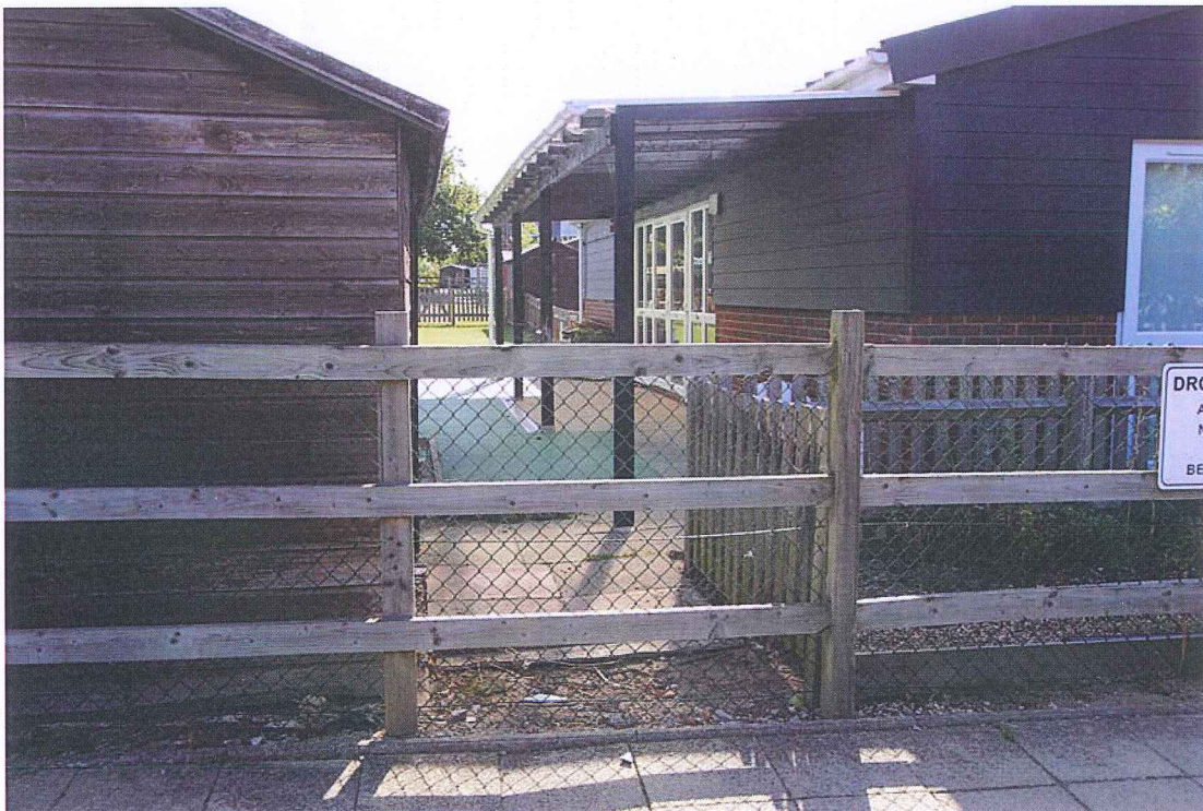
Fig 01 - View of post & rail security fence around existing William Older School Charity owned playgroup building.
