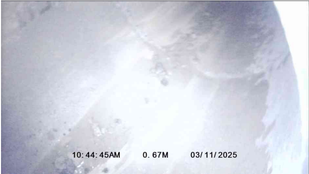
2, 00:00:14, 0.67 m Finish node, major connection without manhole, reference: MAIN
