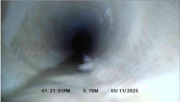
2, 00:00:19, 5.76 m Point repair, localised lining from 12 o'clock to 11 o'clock, start
