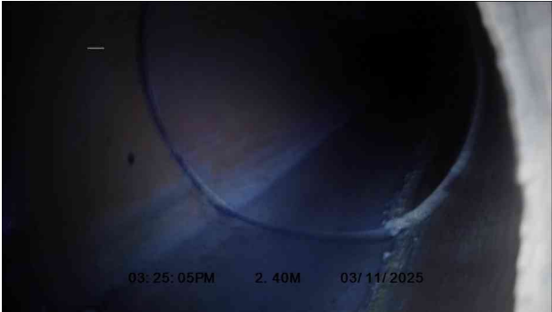
2, 00:00:13, 2.40 m Finish node, major connection without manhole, reference: MAIN
