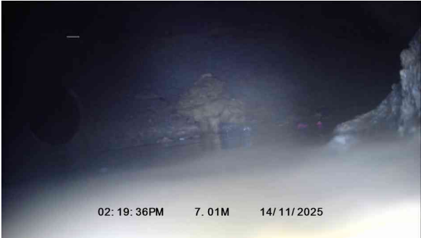
2, 00:00:27, 7.01 m Finish node, manhole, reference: 323A
