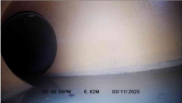
2, 00:00:52, 6.62 m Finish node, major connection without manhole, reference: MAIN
