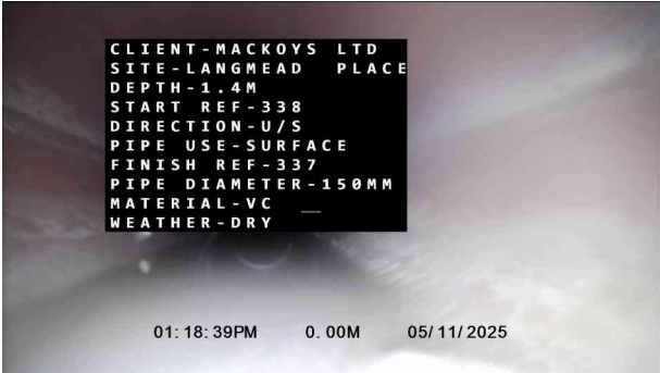
1, 00:00:00, 0.00 m Start node, manhole, reference: 338
