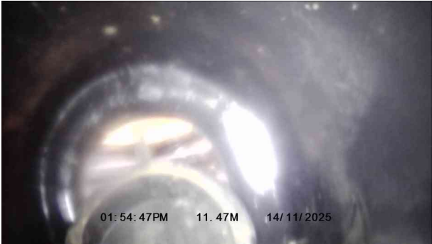
2, 00:00:49, 11.47 m Finish node, gully, reference: RG54
