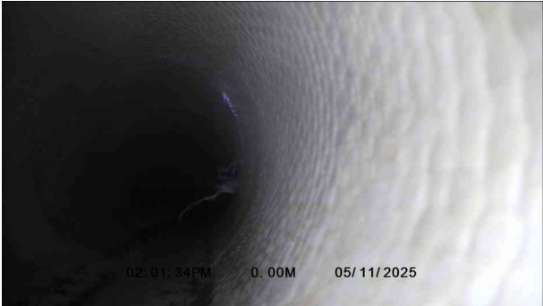
2, 00:00:07, 0.00 m Point repair, localised lining from 12 o'clock to 11 o'clock, start
