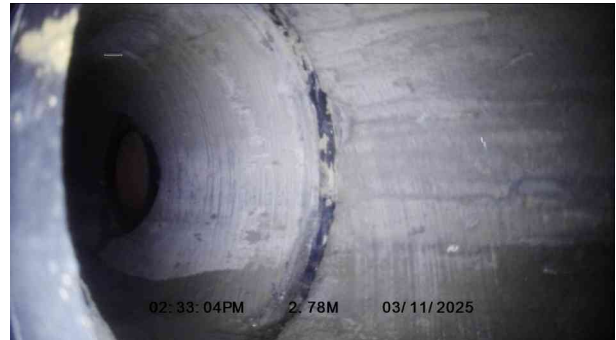
2, 00:00:18, 2.78 m Finish node, major connection without manhole, reference: MAIN
