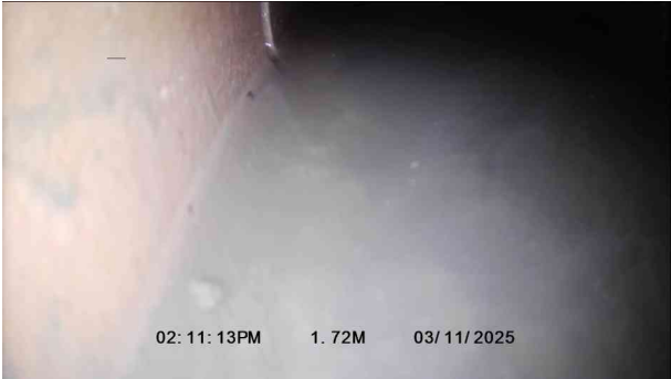
2, 00:00:21, 1.72 m Finish node, major connection without manhole, reference: 264
