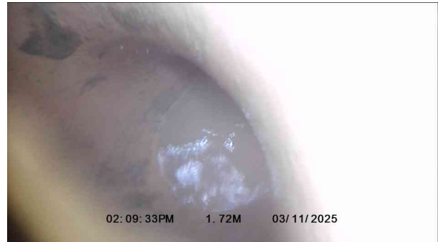
2, 00:00:35, 1.72 m Finish node, major connection without manhole, reference: 264
