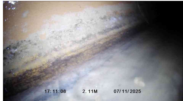
2, 00:00:15, 2.11 m Finish node, major connection without manhole, reference: MAIN
