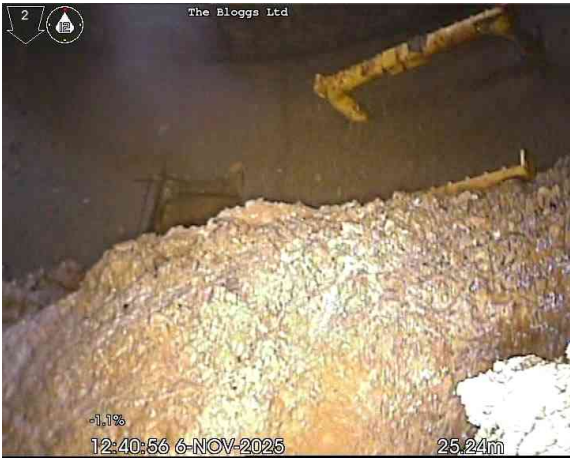
2, 00:02:49, 25.24 m Finish node, manhole, reference: F20
