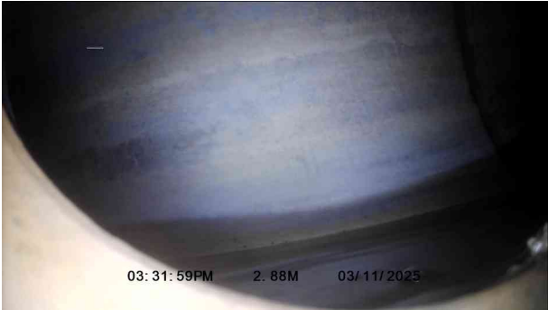
2, 00:00:18, 2.88 m Finish node, major connection without manhole, reference: MAIN
