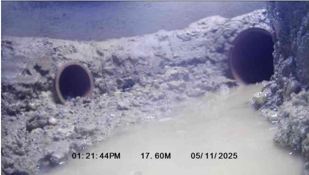
3, 00:01:01, 17.60 m Finish node, manhole, reference: 340
