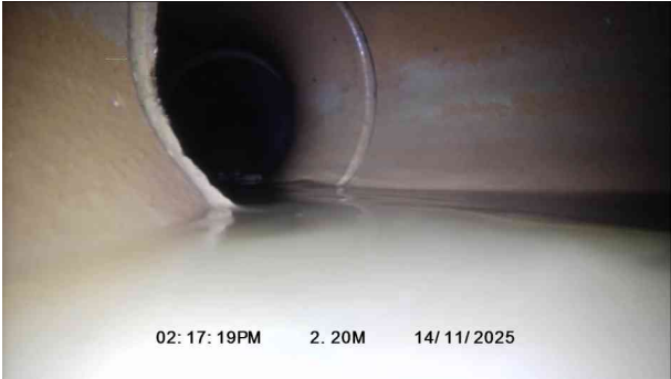
2, 00:00:13, 2.20 m Finish node, major connection without manhole, reference: MAIN
