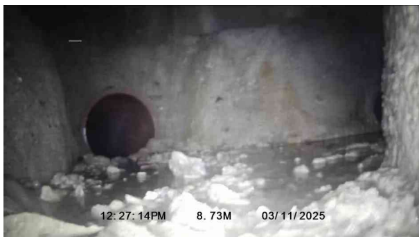
3, 00:00:42, 8.73 m Finish node, manhole, reference: 261
