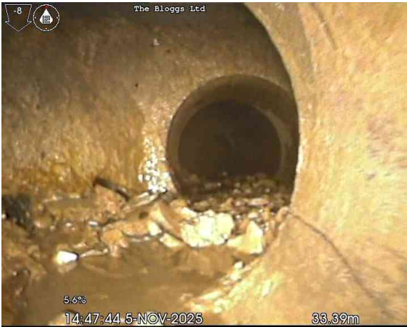
1, 00:03:39, 33.39 m Finish node, manhole, reference: S217
