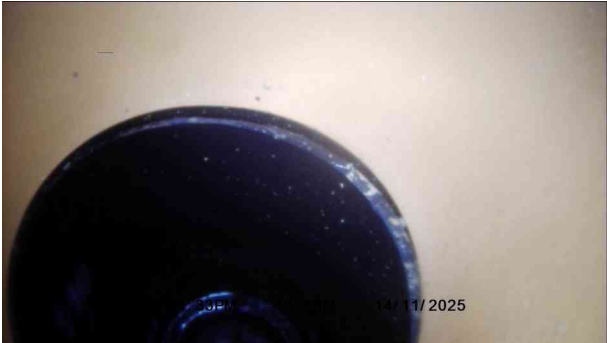
2, 00:01:04, 15.56 m Finish node, gully, reference: RG53
