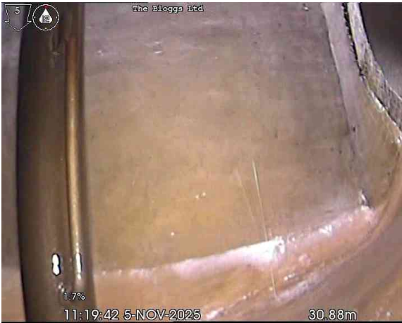
2, 00:03:04, 30.88 m Finish node, manhole, reference: S2706
