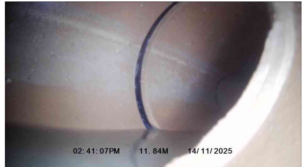
2, 00:00:56, 11.84 m Finish node, major connection without manhole, reference: MAIN
