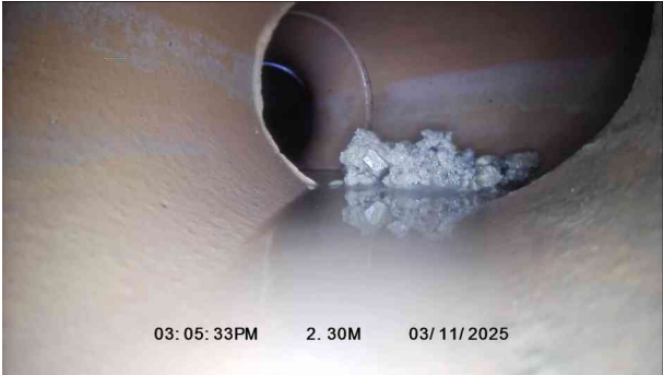
2, 00:00:37, 2.30 m Finish node, major connection without manhole, reference: MAIN
