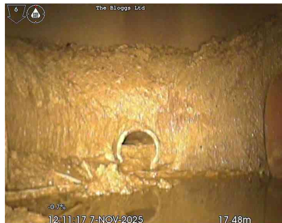
2, 00:01:28, 17.48 m Finish node, manhole, reference: 323A
