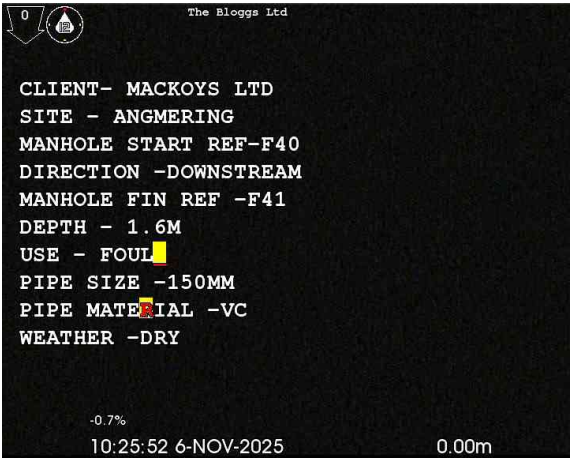
1, 00:00:00, 0.00 m Start node, manhole, reference: F40
