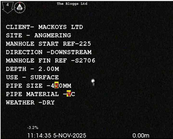
1, 00:00:00, 0.00 m Start node, manhole, reference: 225
