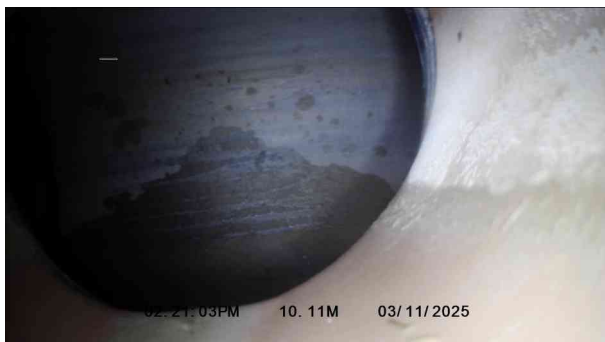
3, 00:00:23, 10.11 m Finish node, major connection without manhole, reference: MAIN
