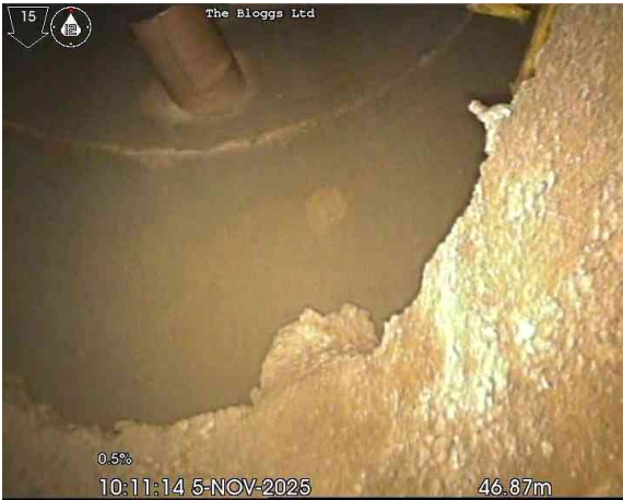
2, 00:04:15, 46.87 m Finish node, manhole, reference: 222
