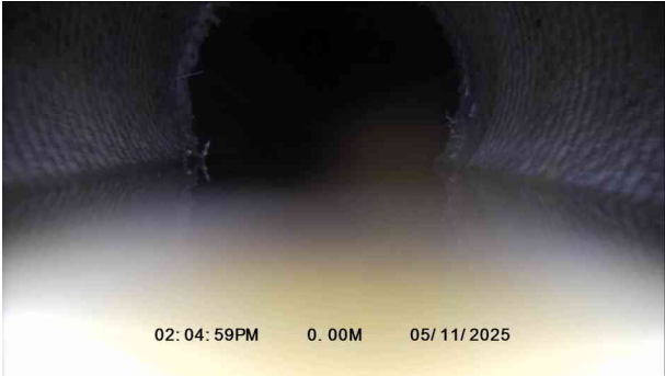
2, 00:00:08, 0.00 m Point repair, localised lining from 12 o'clock to 11 o'clock, start
