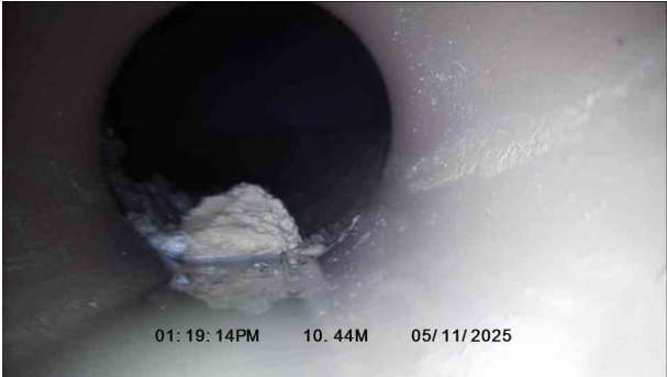
2, 00:00:38, 10.44 m Finish node, manhole, reference: 337
