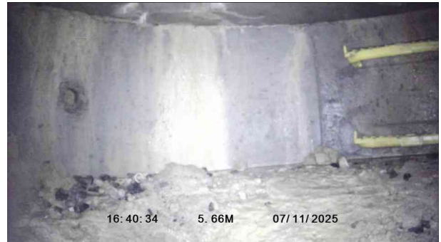
2, 00:00:36, 5.66 m Finish node, manhole, reference: F18
