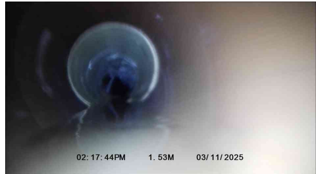
2, 00:00:18, 1.53 m Point repair, localised lining from 12 o'clock to 11 o'clock, start
