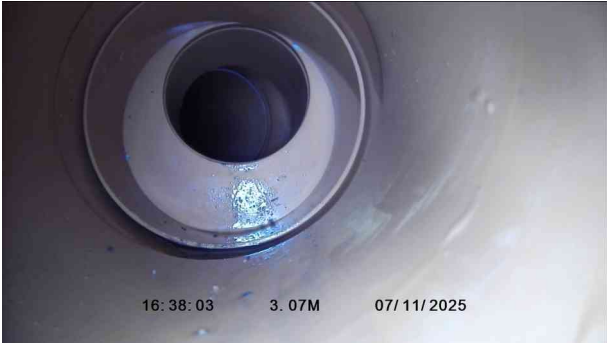
3, 00:01:02, 3.07 m Finish node, manhole, reference: FW230
