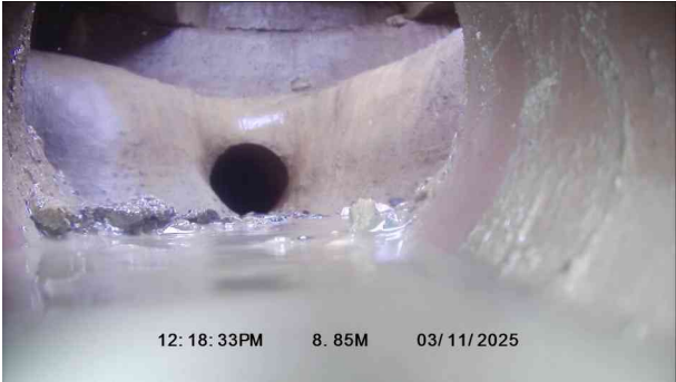
2, 00:00:34, 8.85 m Finish node, manhole, reference: 262
