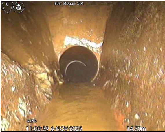
2, 00:01:59, 14.70 m Finish node, manhole, reference: F43
