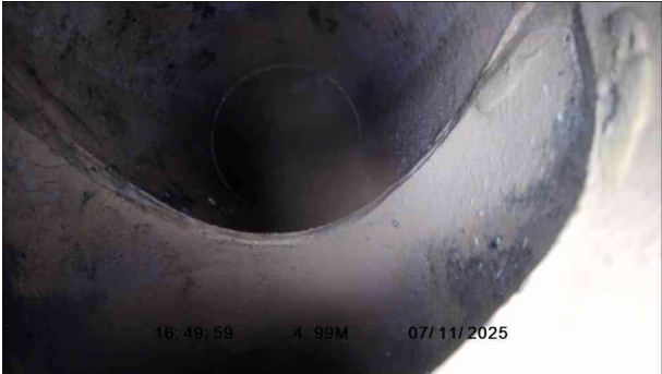
2, 00:00:31, 4.99 m Finish node, manhole, reference: F39
