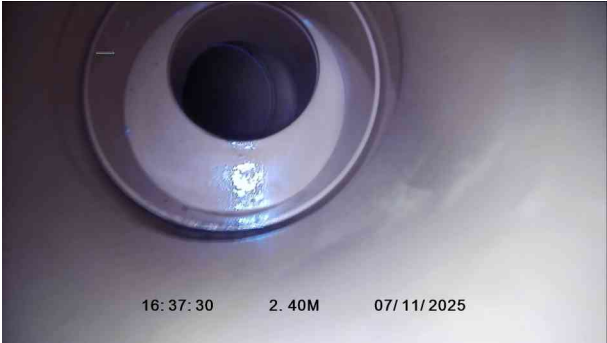
2, 00:00:28, 2.40 m Pipe size changes, new size(s), 100mm high
