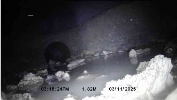
2, 00:00:15, 1.82 m Finish node, manhole, reference: 340
