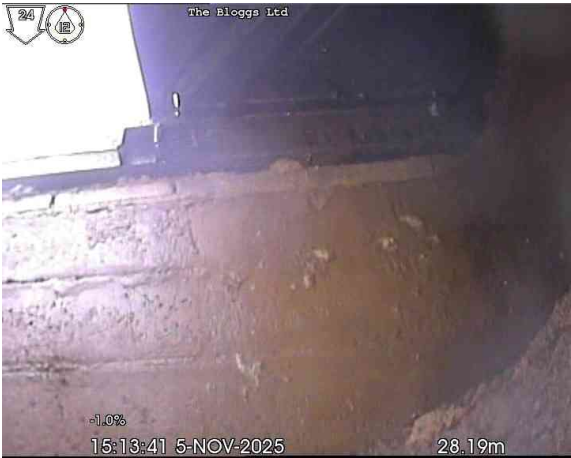
2, 00:02:13, 28.19 m Finish node, manhole, reference: 324
