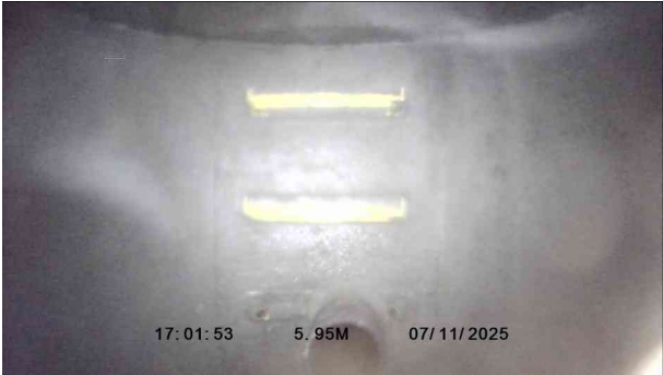
2, 00:00:25, 5.95 m Finish node, manhole, reference: F41
