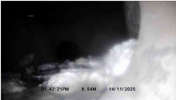
3, 00:00:23, 8.54 m Finish node, manhole, reference: 261
