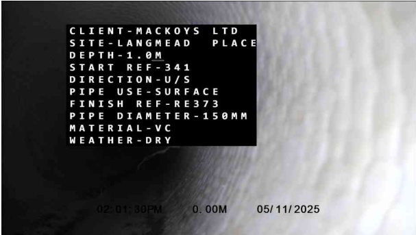
1, 00:00:00, 0.00 m Start node, manhole, reference: 341
