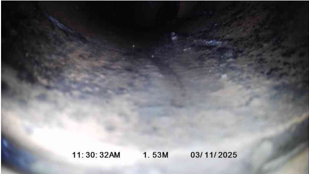
2, 00:00:31, 1.53 m Finish node, major connection without manhole, reference: MAIN
