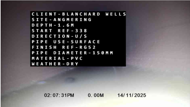
1, 00:00:00, 0.00 m Start node, gully, reference: 338
