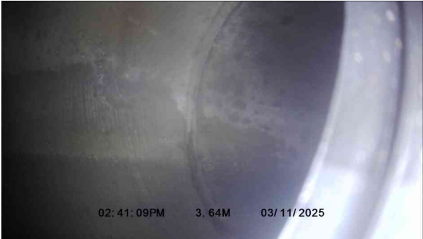
2, 00:00:18, 3.64 m Finish node, major connection without manhole, reference: MAIN
