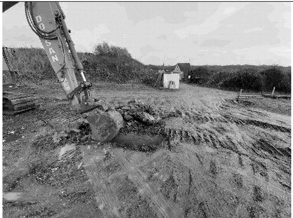
MTP341: Showing trial hole location.
