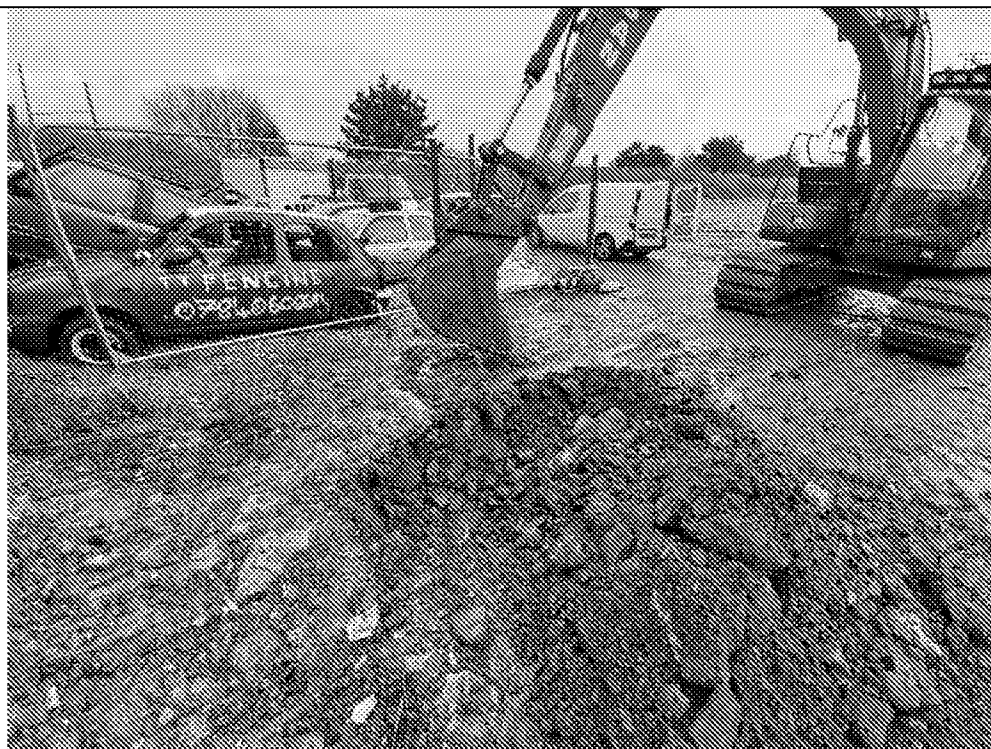
MTP335: Showing trial hole location.
