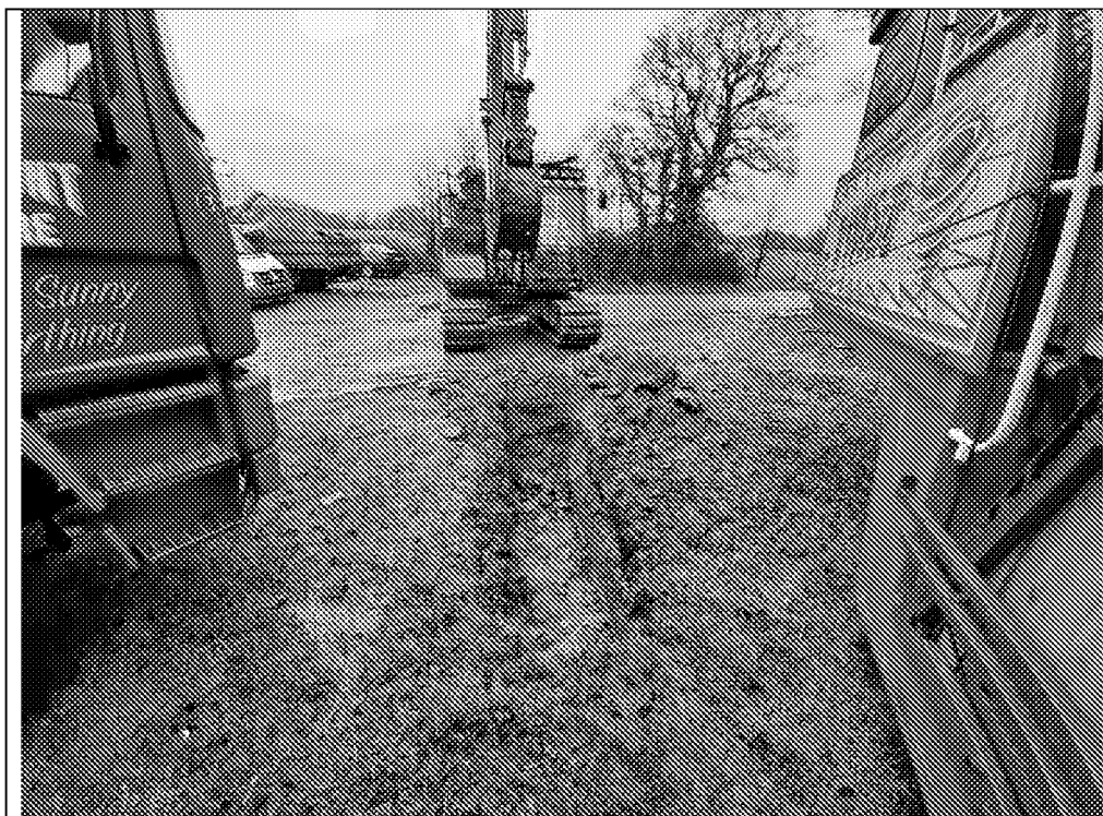
MTP339: Showing trial hole location.
