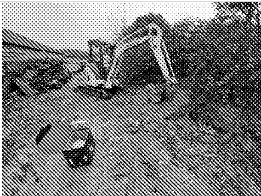
MTP337: Showing trial hole location (into bund).
