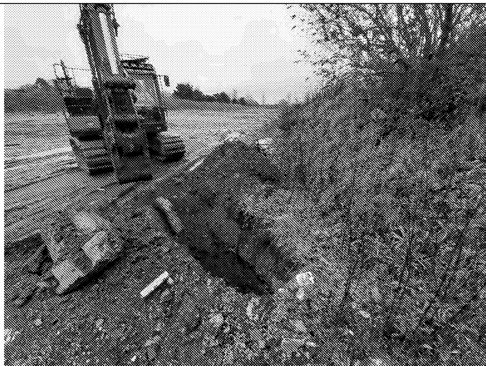
MTP336: Showing trial hole location.
