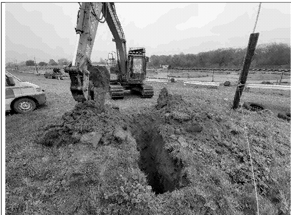
MTP316: Showing trial hole location.
