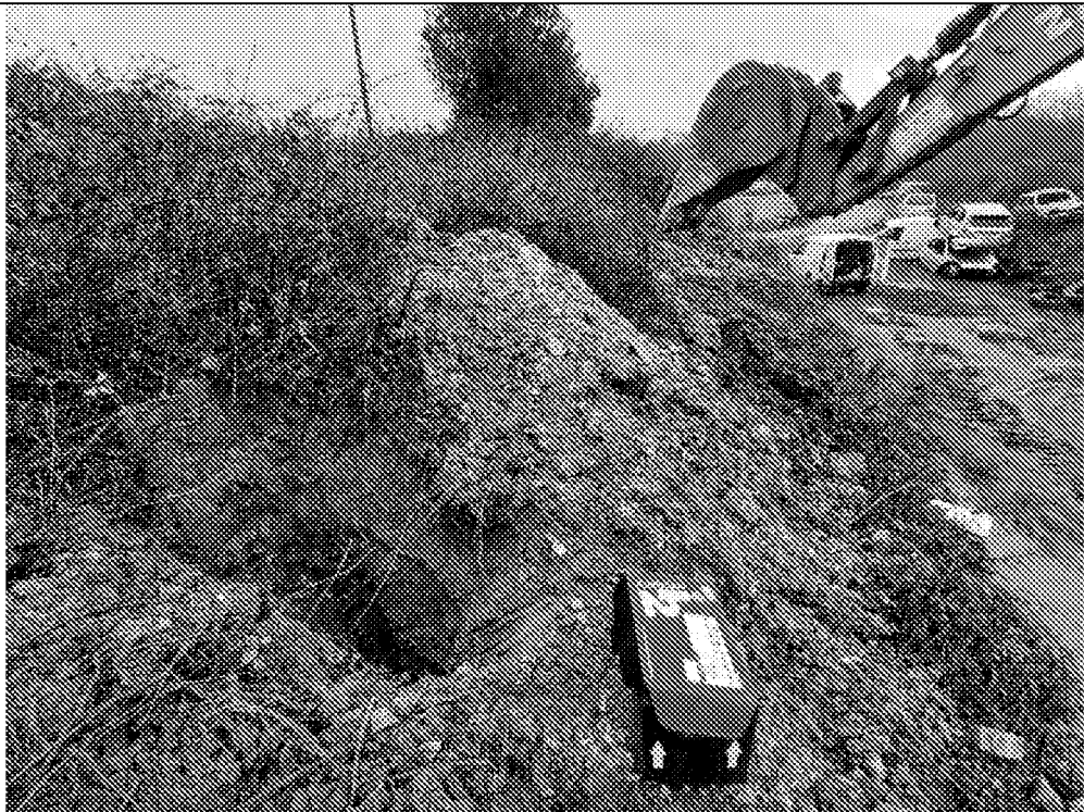
MTP313: Showing trial hole location.
