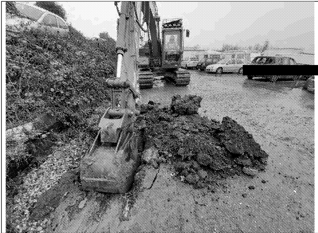
MTP317: Showing trial hole location.
