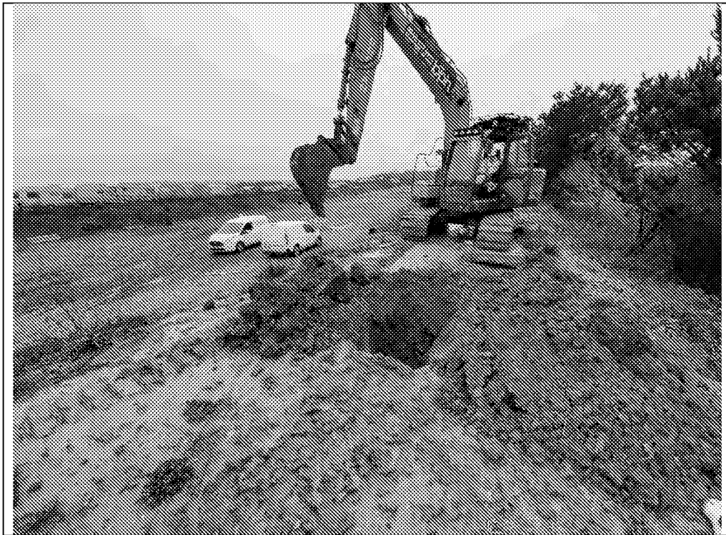
MTP328: Showing trial hole location (on bund).
