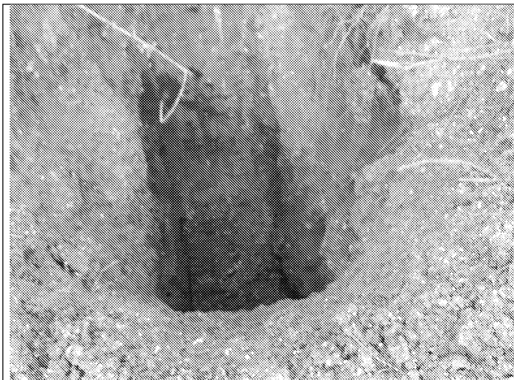
MTP324: Trial hole (into bund).
