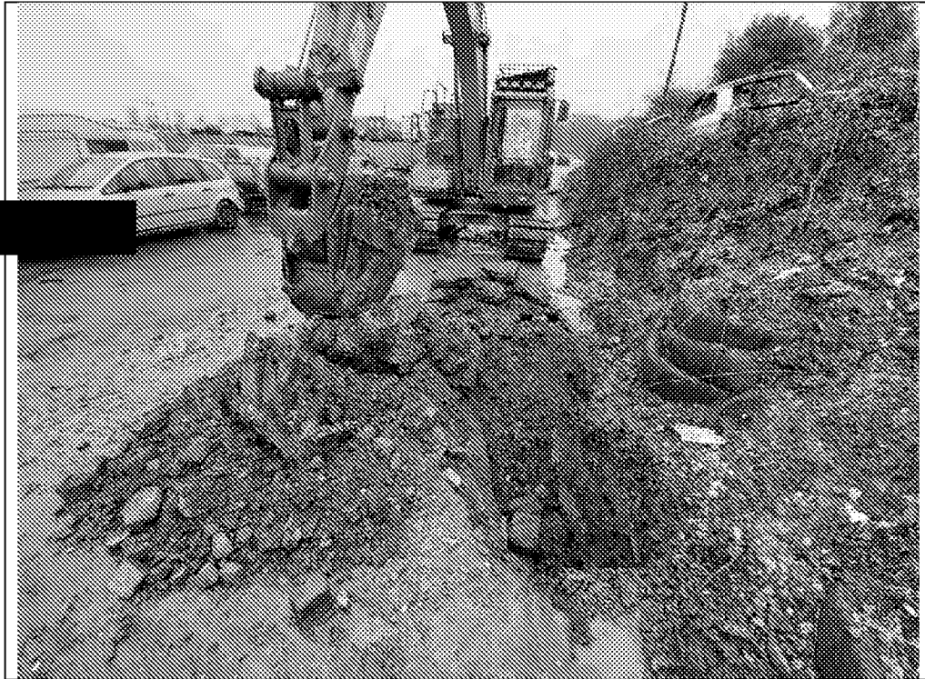
MTP318: Showing trial hole location.
