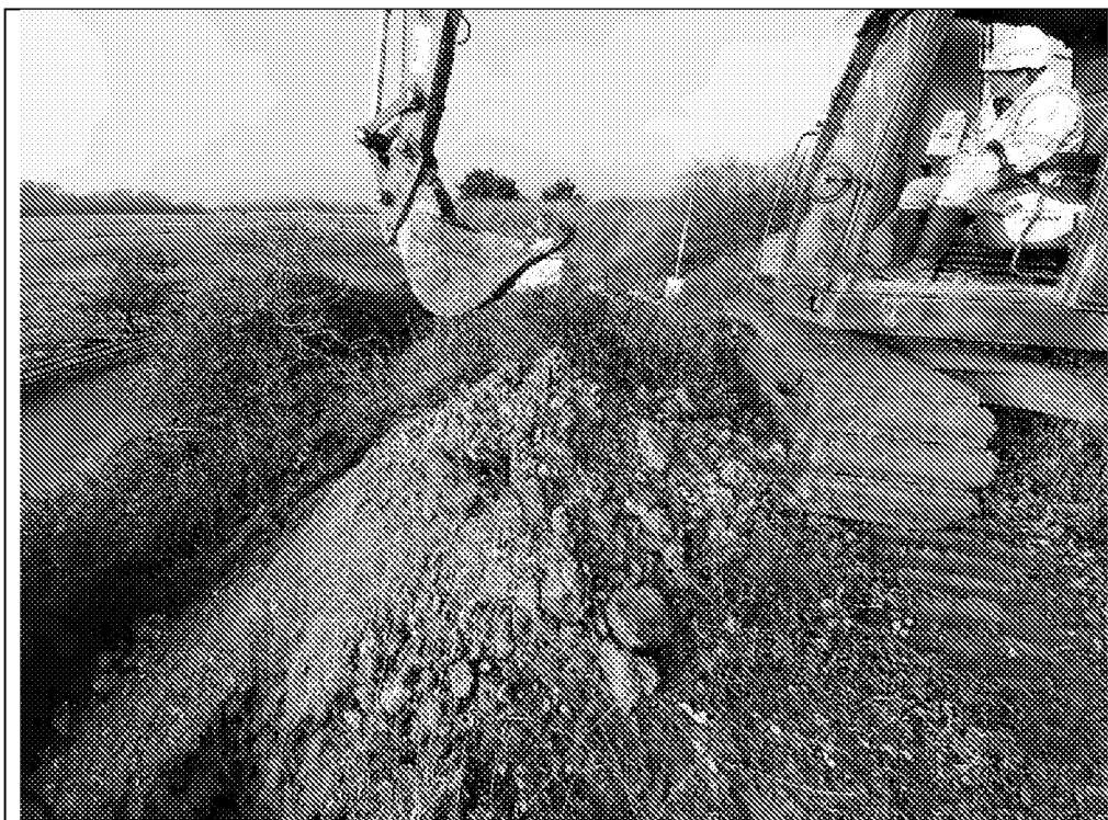
MTP322: Showing trial hole location (on bund).
