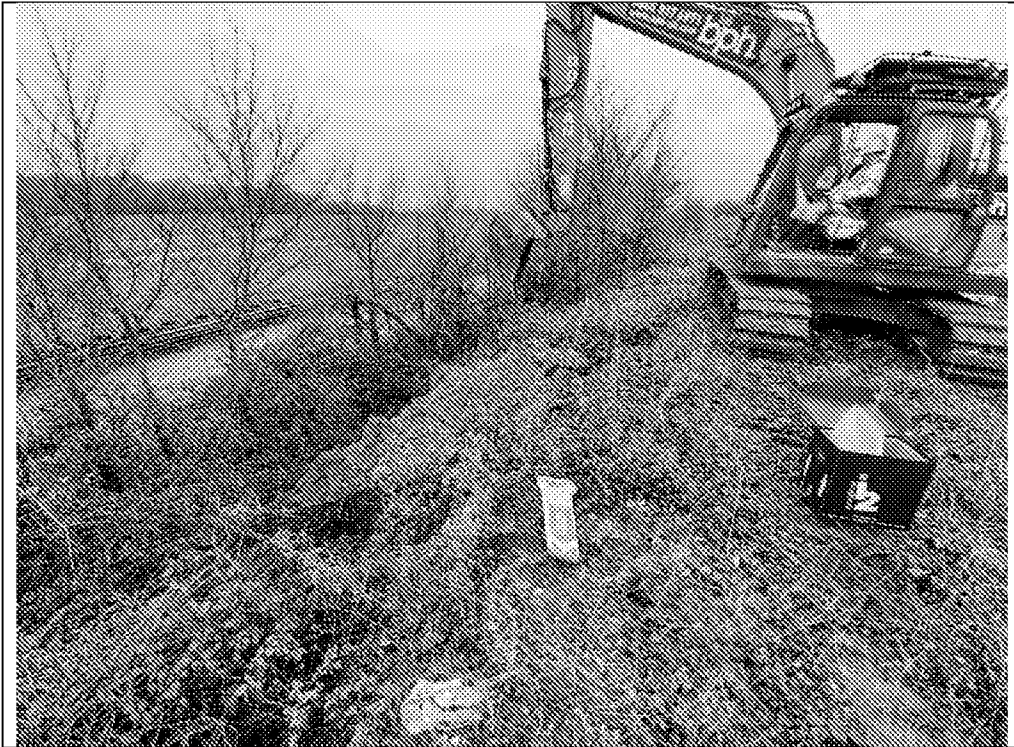
MTP320: Showing trial hole location (on bund).
