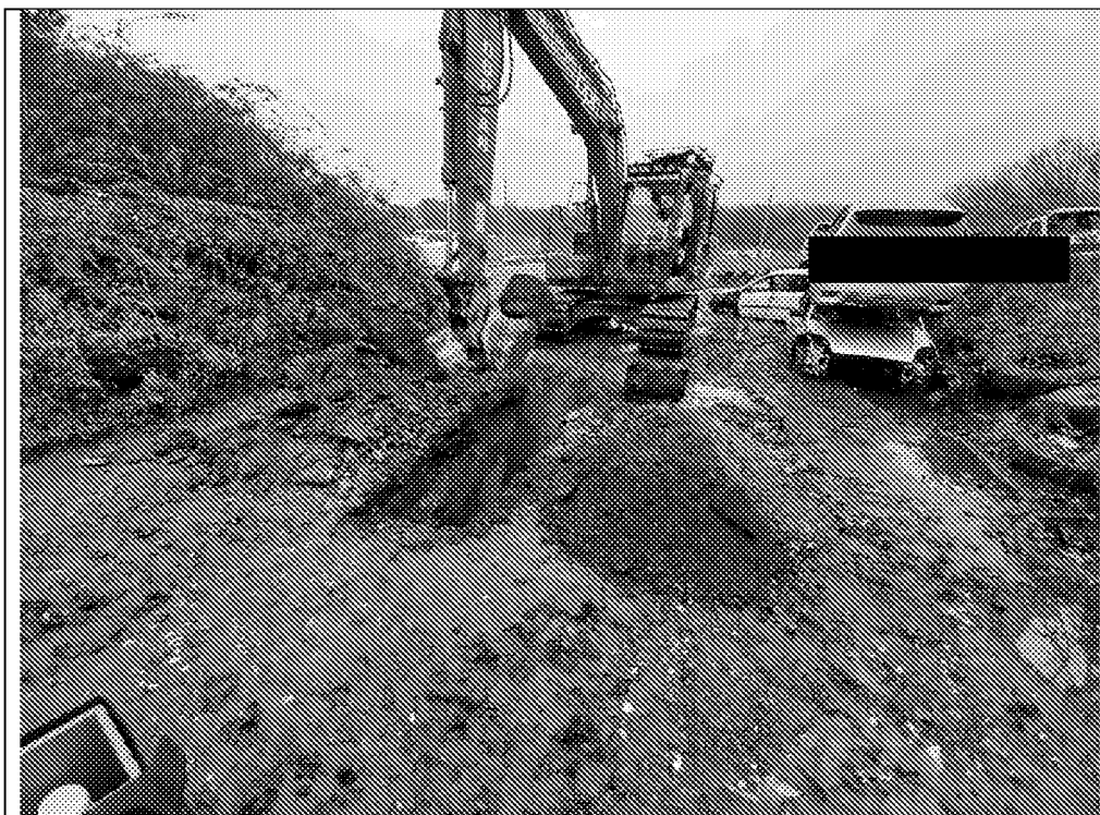
MTP310: Showing trial hole location.
