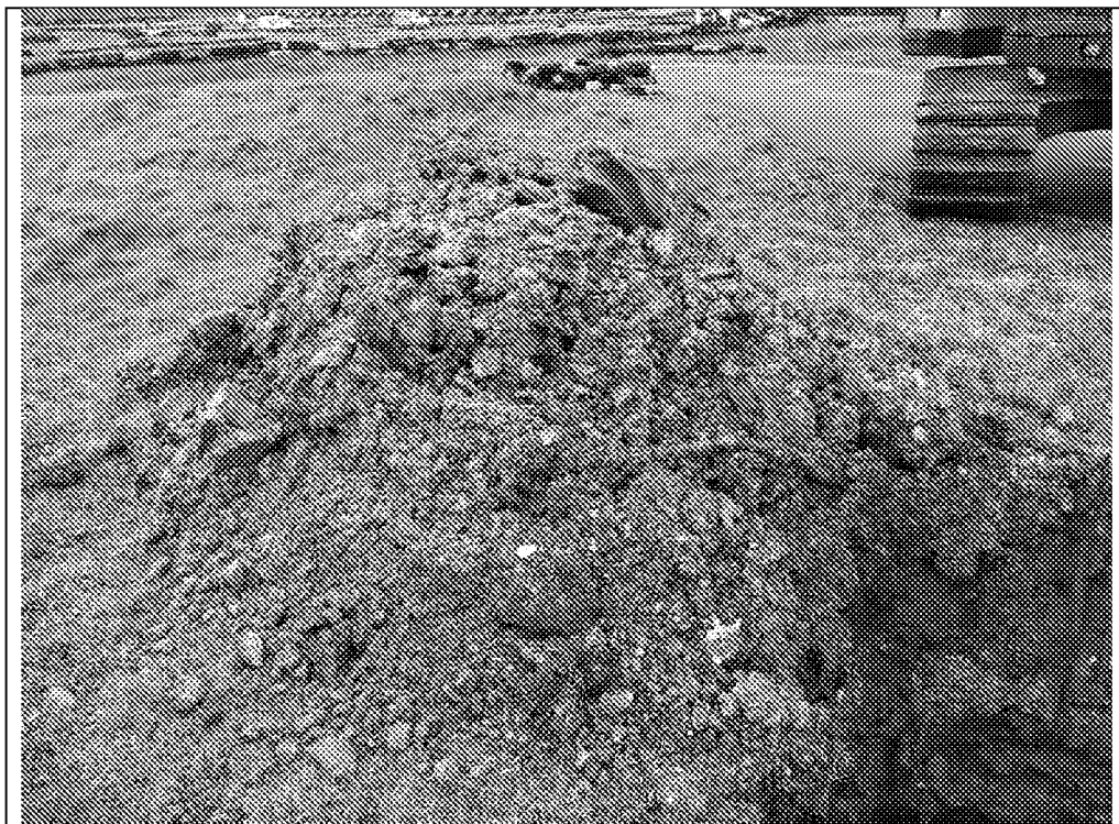
MTP302: Made ground arisings in the raceway area.
