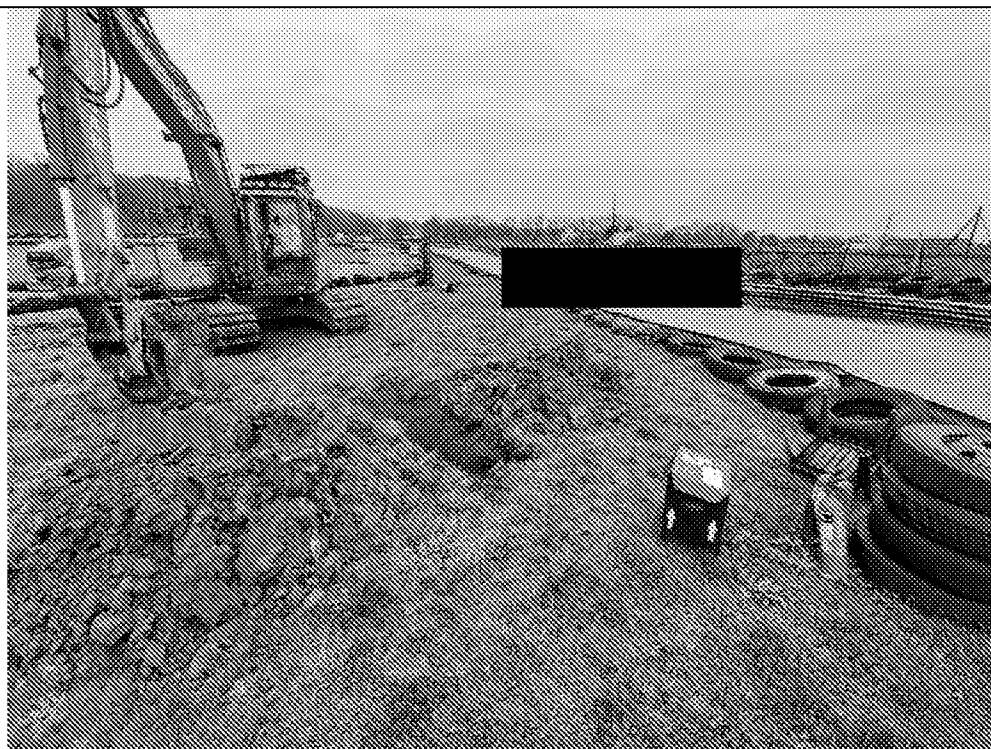
MTP303: Showing trial hole location.
