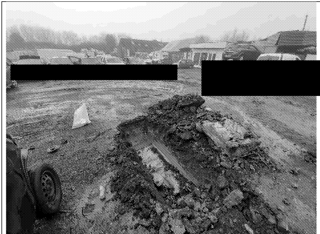
MTP343: Showing trial hole location and arisings.
