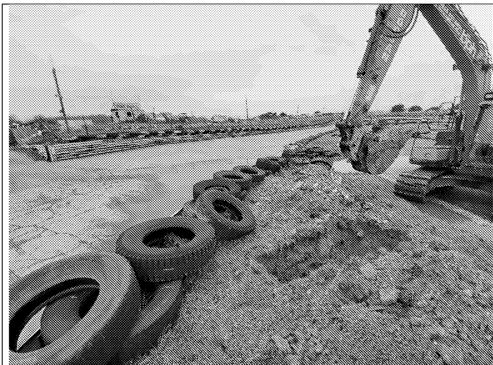
MTP305: Showing trial hole location.
