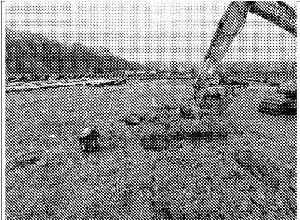
MTP304: Showing trial hole location.
