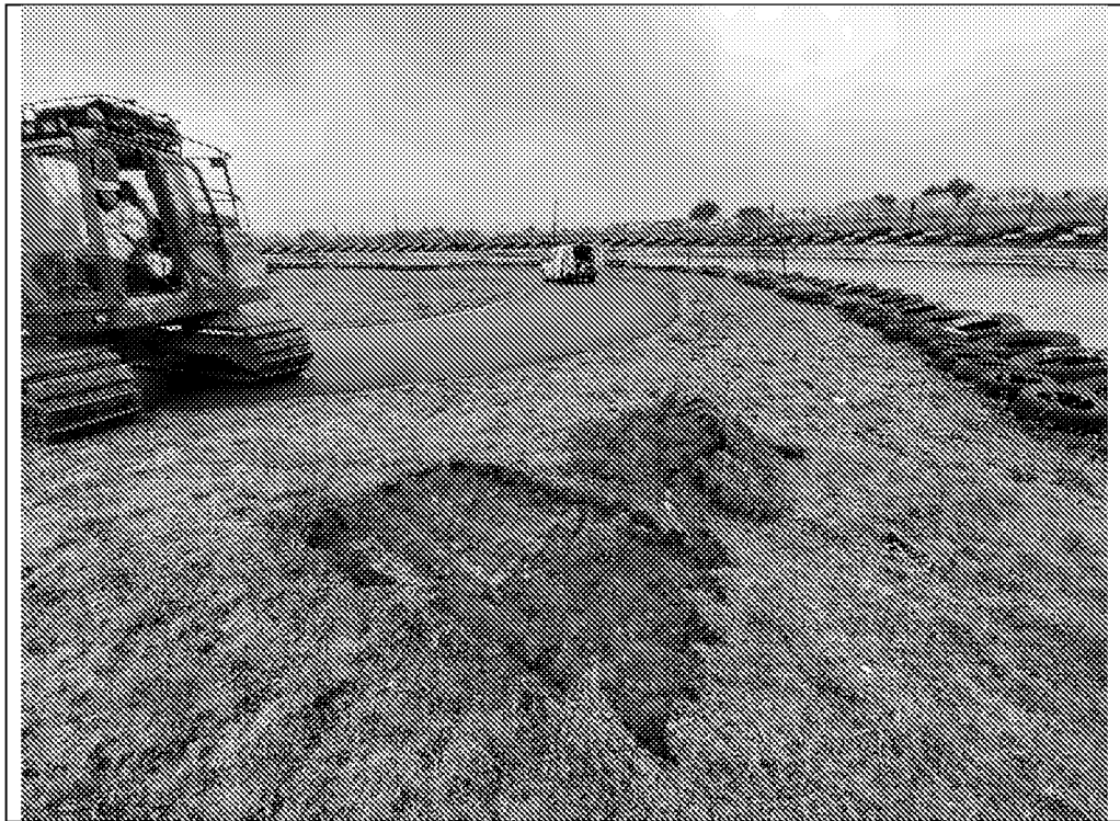
MTP302: Showing trial hole location.
