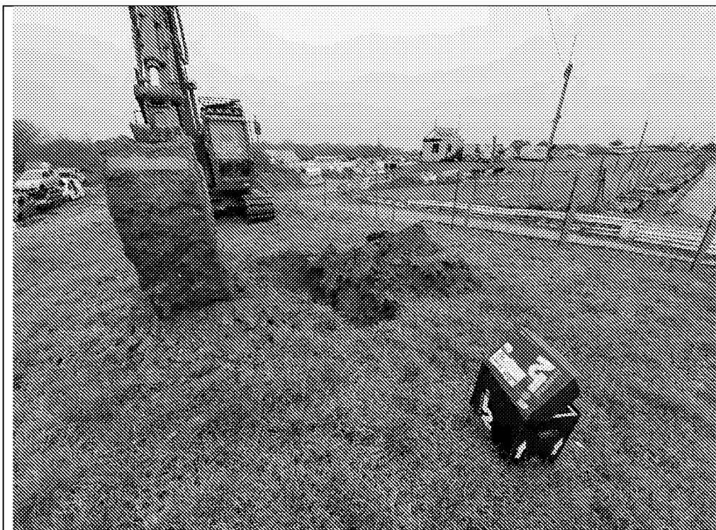
MTP308: Showing trial hole location.
