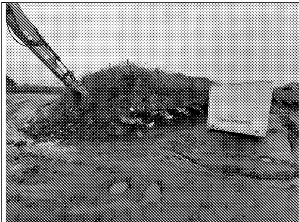
MTP323: Showing trial hole location (into bund).
