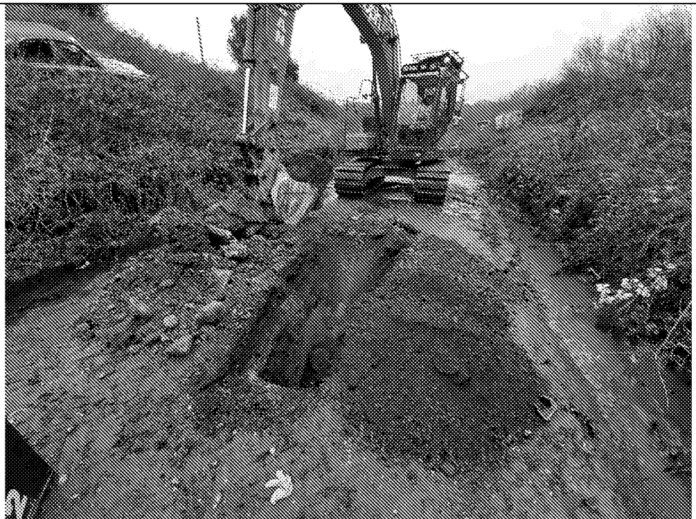
MTP309: Showing trial hole location.
