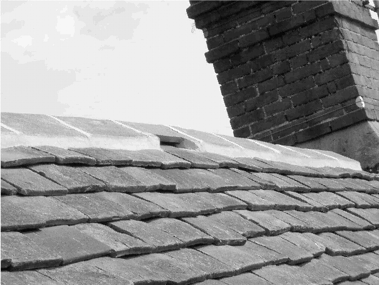
Example of access point under ridge tile
