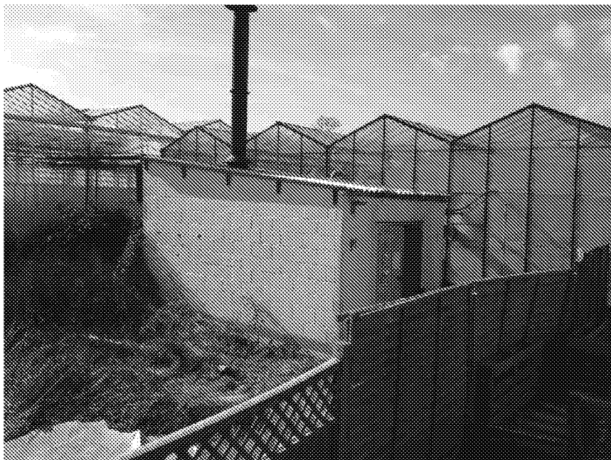
Plant room on the east of the site.
