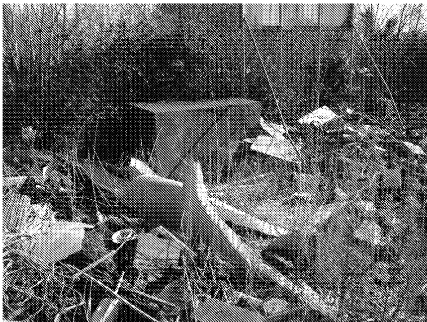
Demolition spoil and above ground oil tank formerly located in the plant room.
