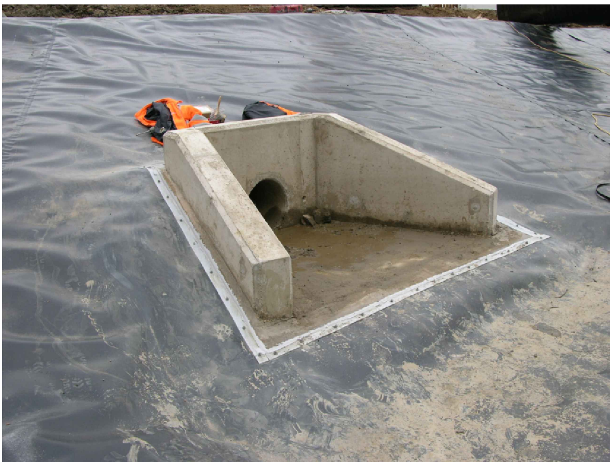
Example Headwall Liner Sealing Detail
