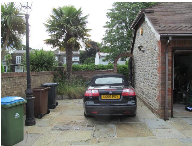
Front View Existing Garage
