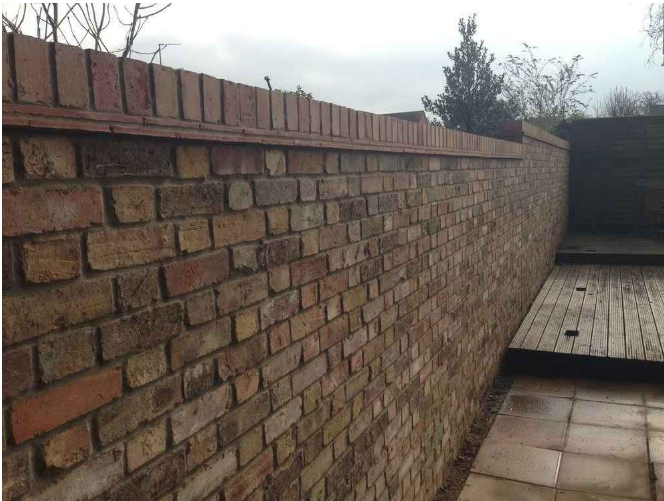
1.8m brick wall with tile crease top
