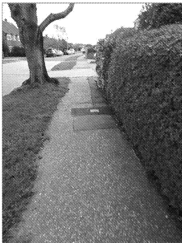
Footway on Shardeloes Road
