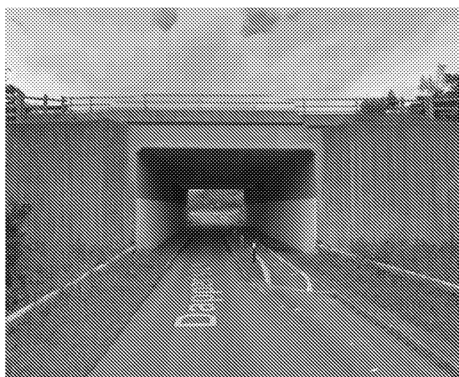
Figure 3.4: Narrow Carriageway Under the Bridge
