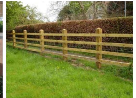
Fencing around the LEAP: Post and rail fence with netting, 1.2m high
