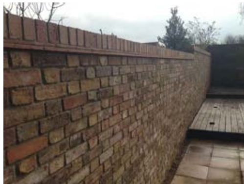
1.8m brick wall with tile crease top
