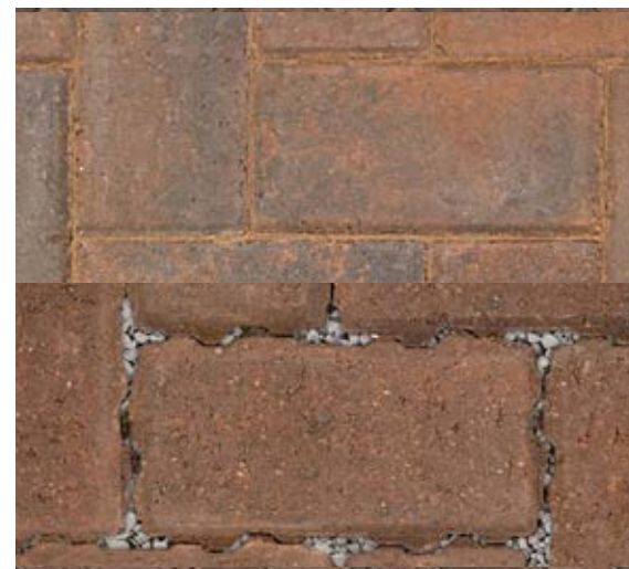
Block paving: [refer to the landscape plans] Supplier: Marshall; Product: MARSHALLS KEYBLOK BURNT OCHRE & MARSHALLS PRIORA BURNT OCHRE
