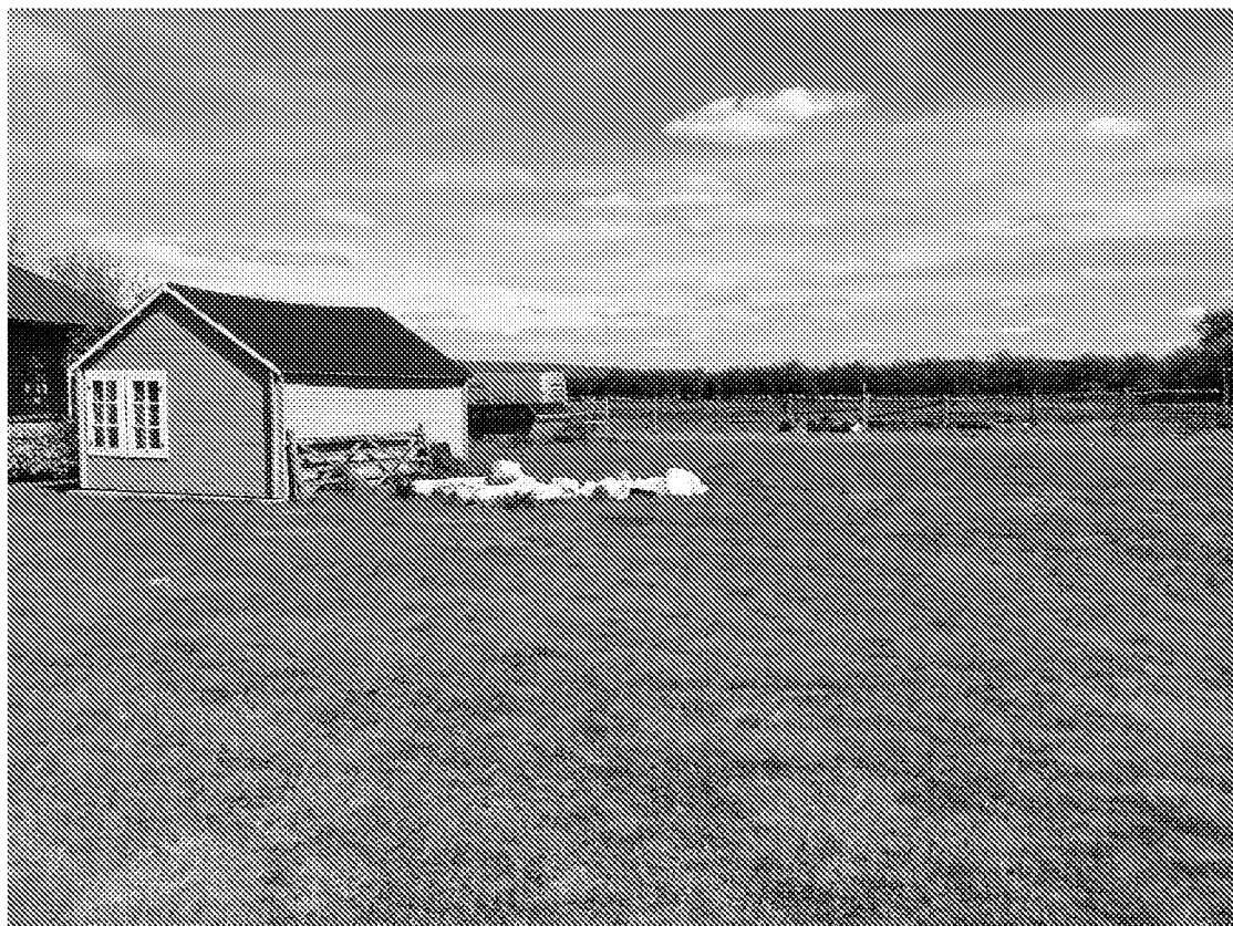
Figure 4. Wooden building surrounded by short amenity grass.
