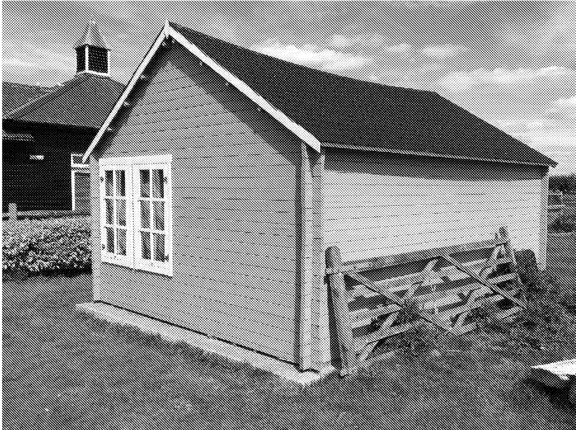
Figure 7. South and west faces of Shiplap building with no roof void and bitumen tiles for the roof.
