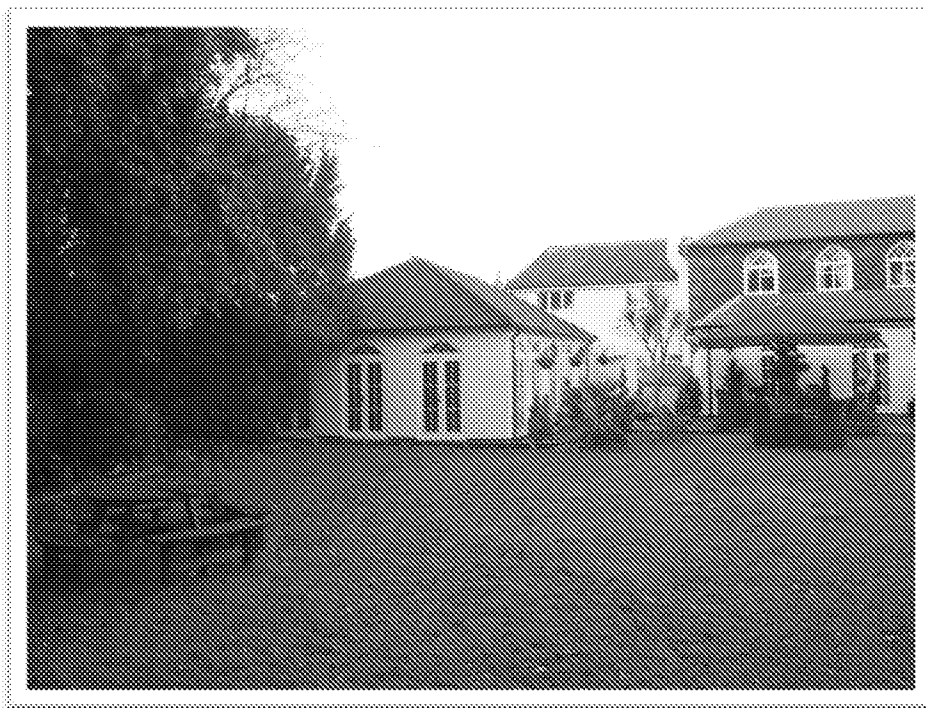
Photograph 1:- The site of the proposed building within the rear garden
