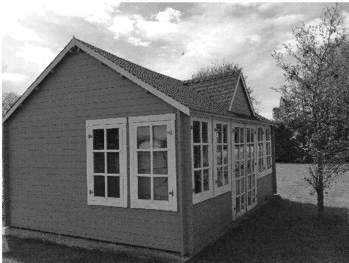
Figure 8. North and east faces of shiplap building.
