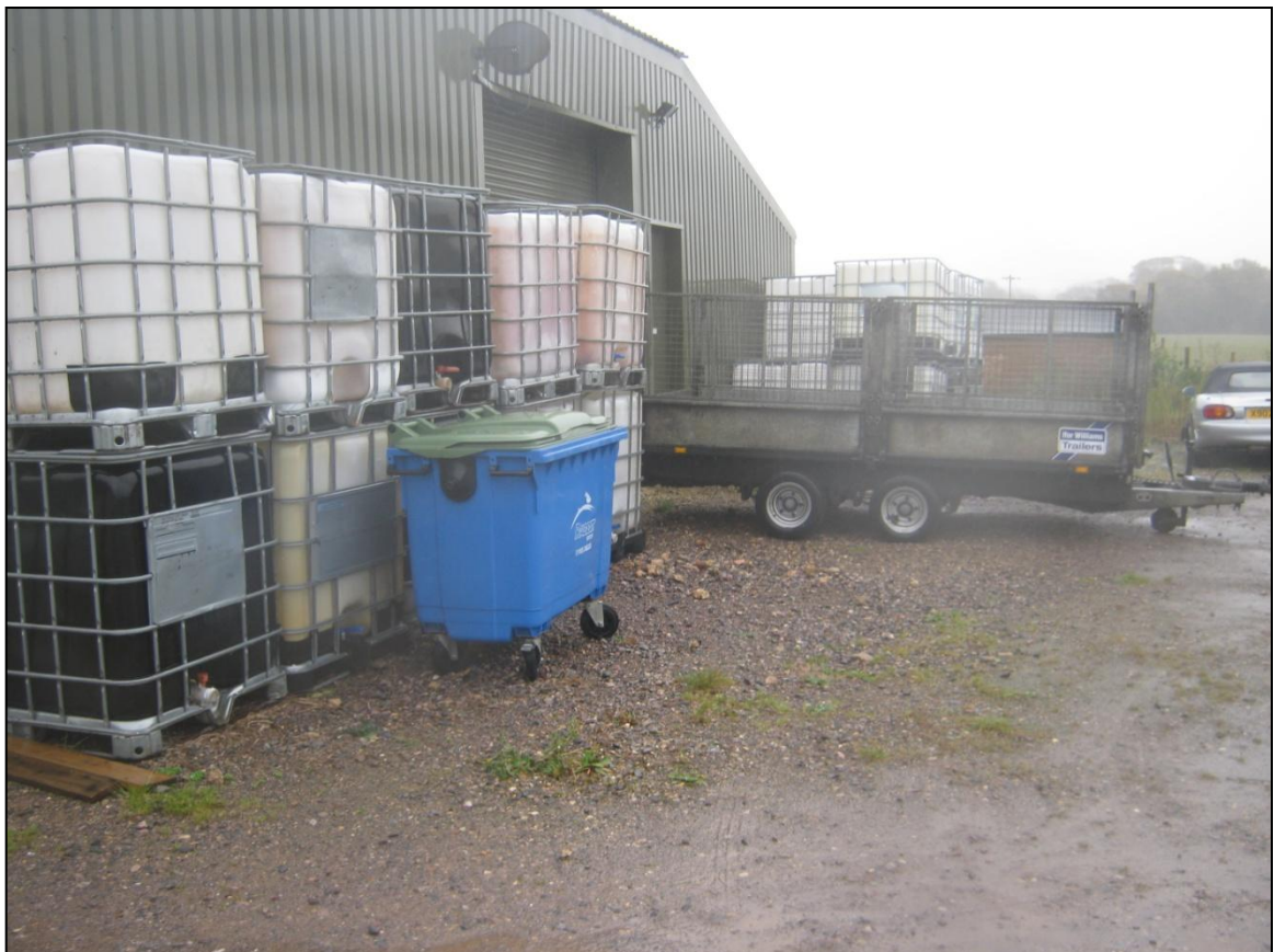
Warehouse Building used to Store Stage Props and Empty Plastic Containers
