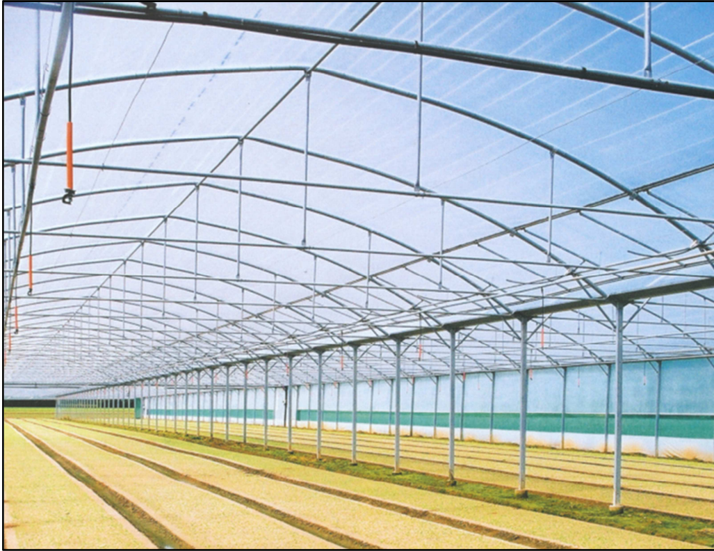
Fig 6. The inside of the covered storage showing the construction.
