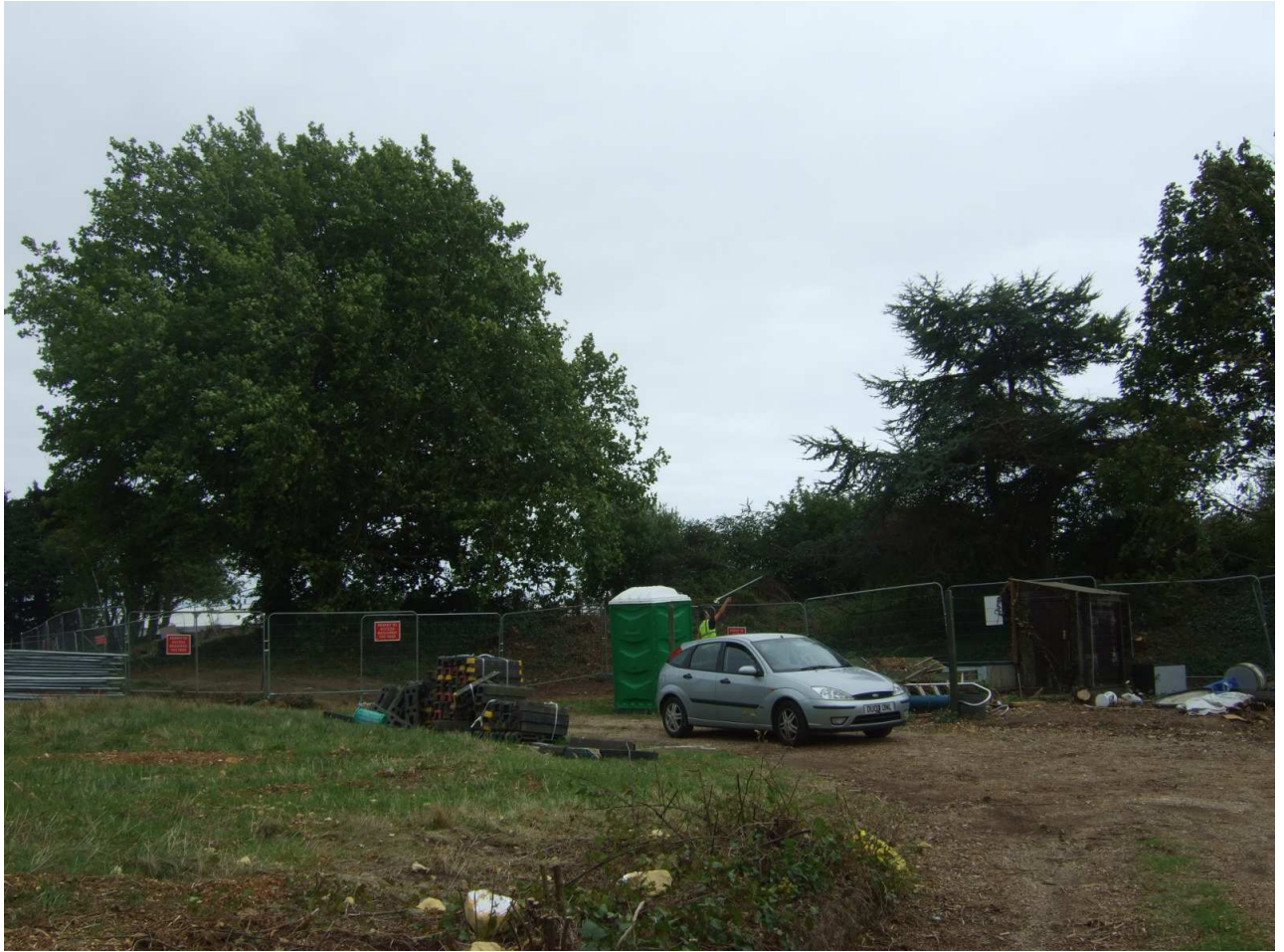
Fig.5 Looking SE towards T53 and T54
