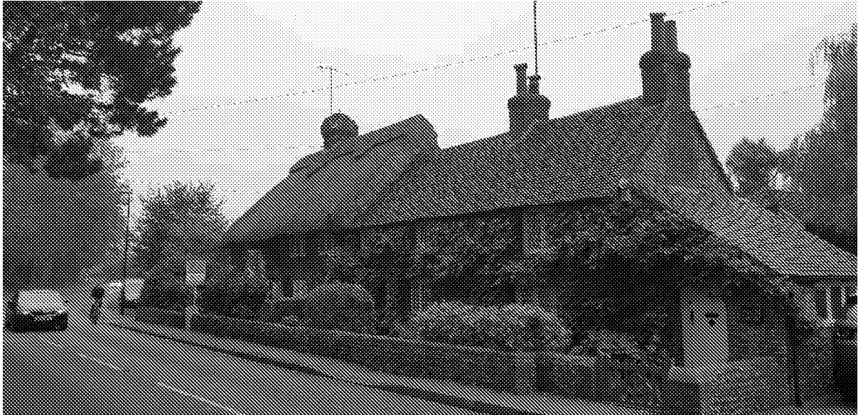
Photograph showing The Old Cottage viewed from the South West. Refer to Drawing 19068 for proposed works.
