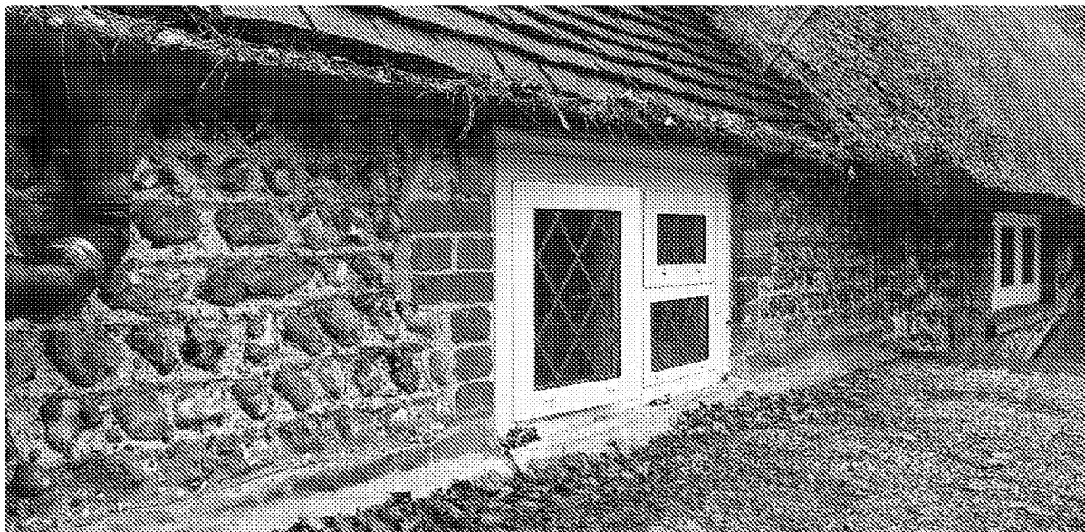
Photograph showing the first floor bathroom window cill which requires replacing. See note 08 on drawing 19068 2.01.
