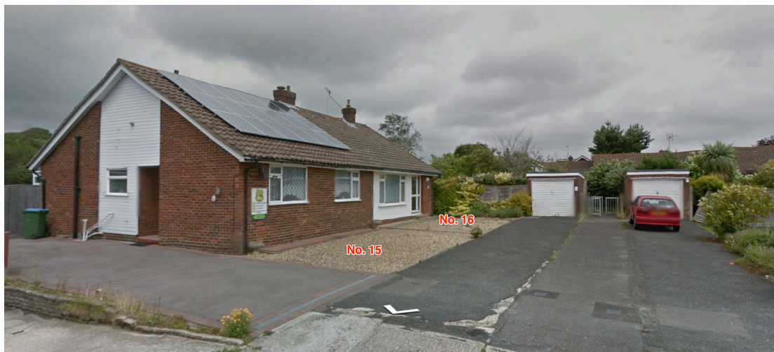
View from street at Nos. 15 and 16 (application property)
