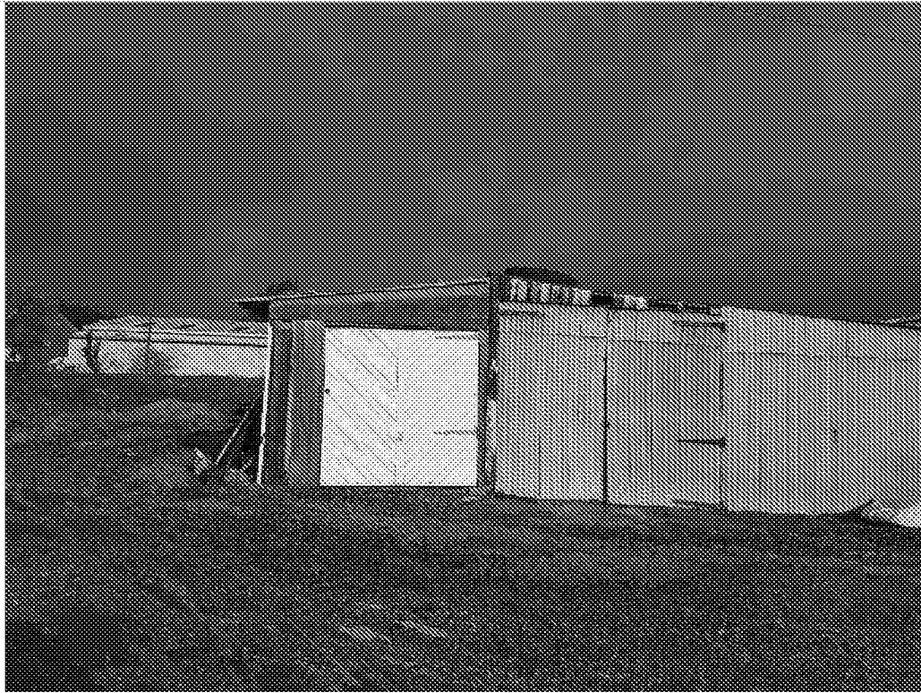
Plate 5 -- Sheds in the north western corner of the site.
