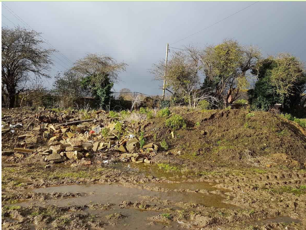
Plate 4 – Building rubble and ear stockpiles along the site's western boundary.
