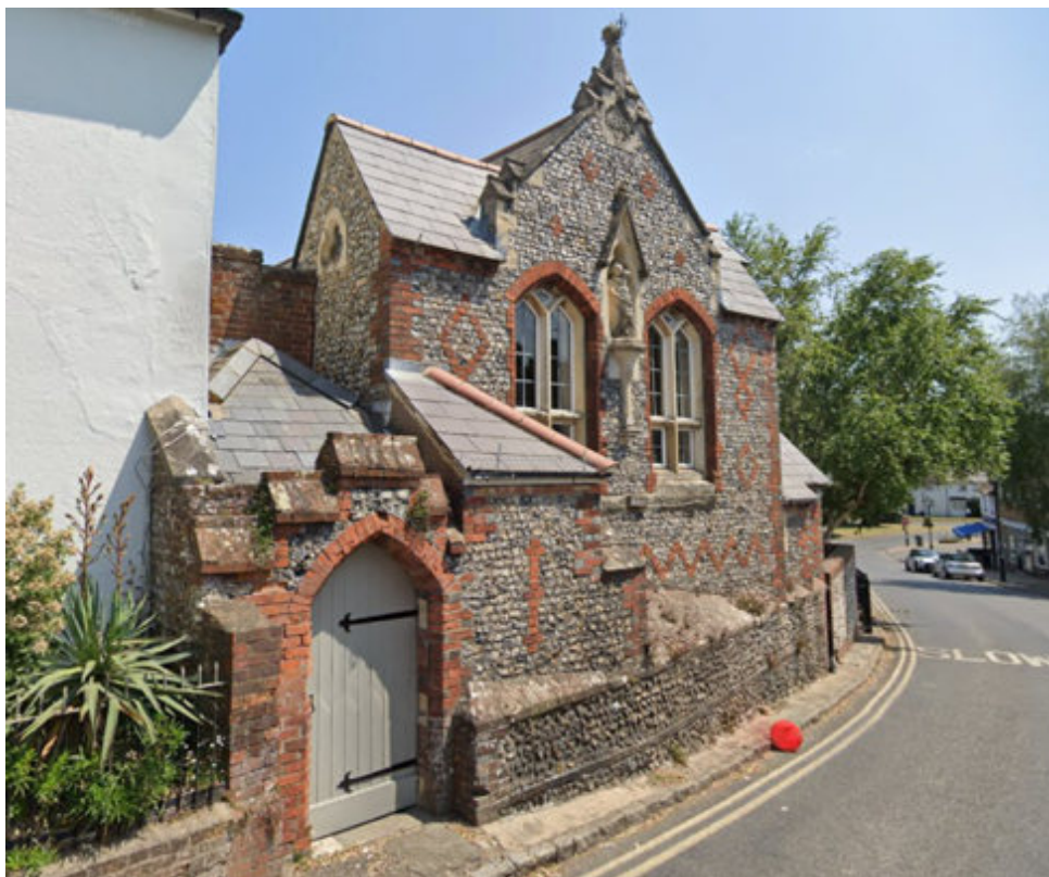
The former Master's house with diapered brickwork and flint laid to course. (© Google)
