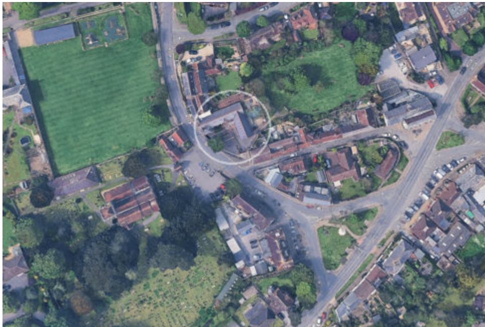
Aerial view of Angmering Village with the library highlighted. © Google
