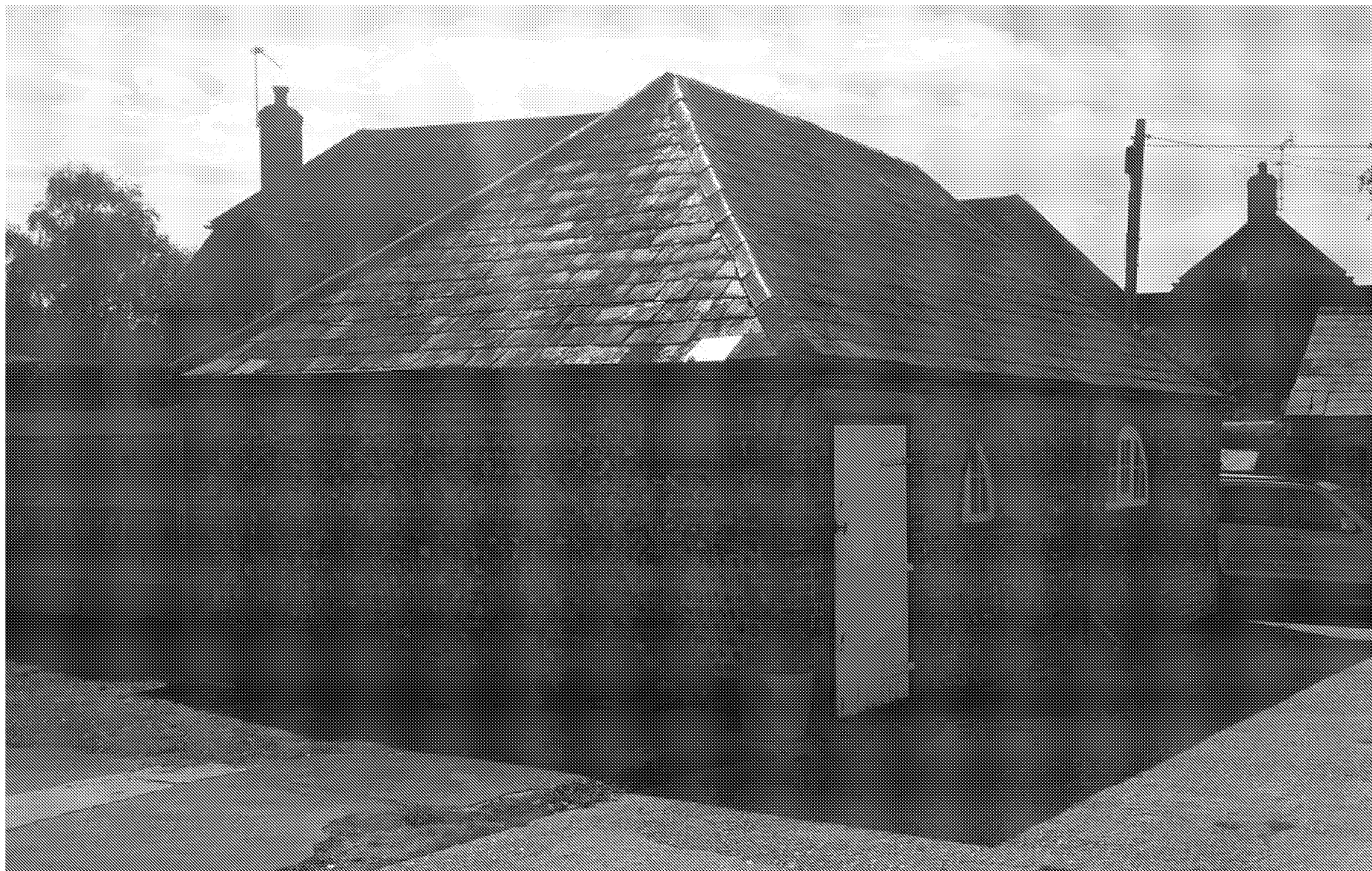
External view of Building 2
