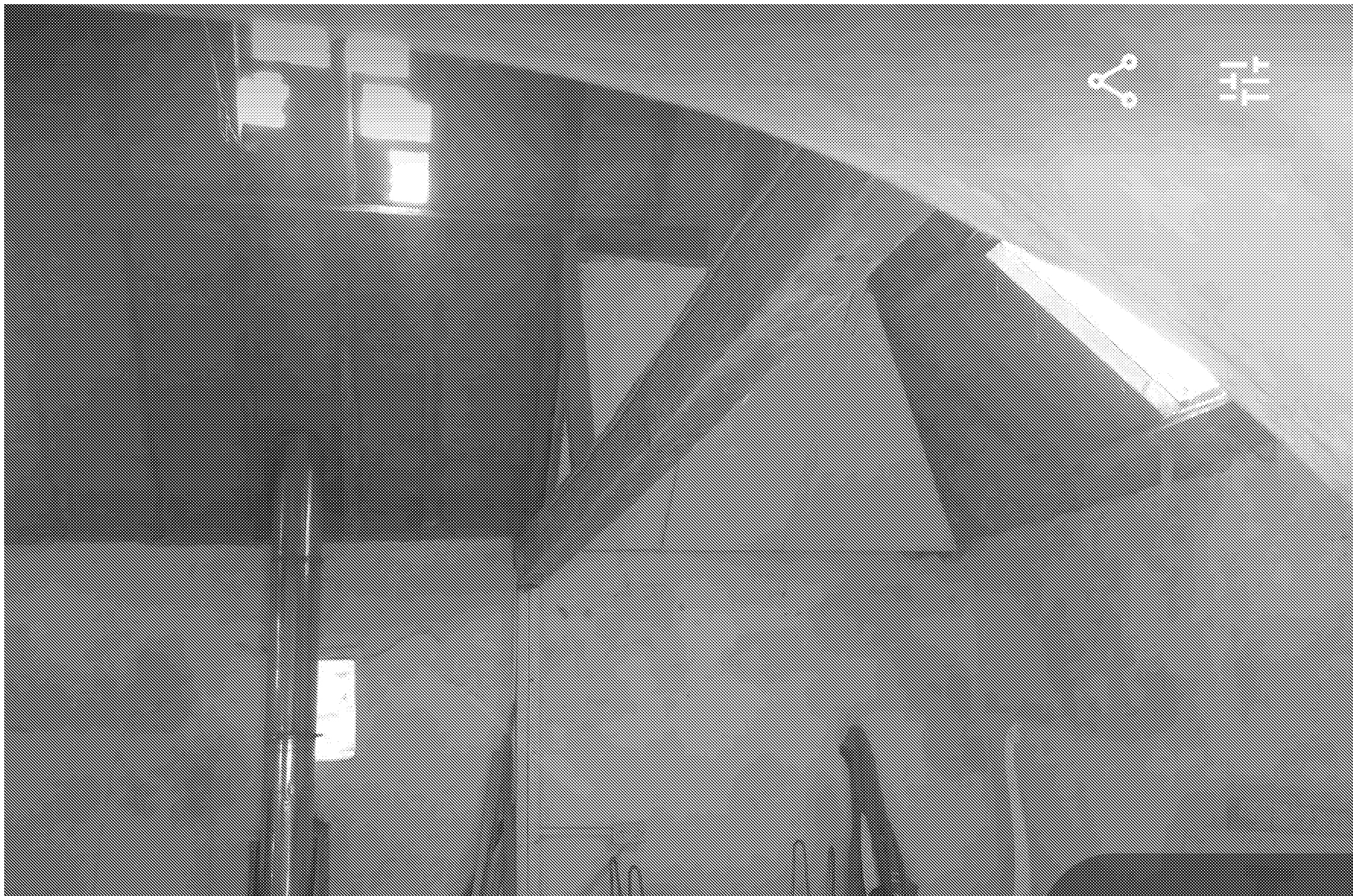
Internal view of Building 2
