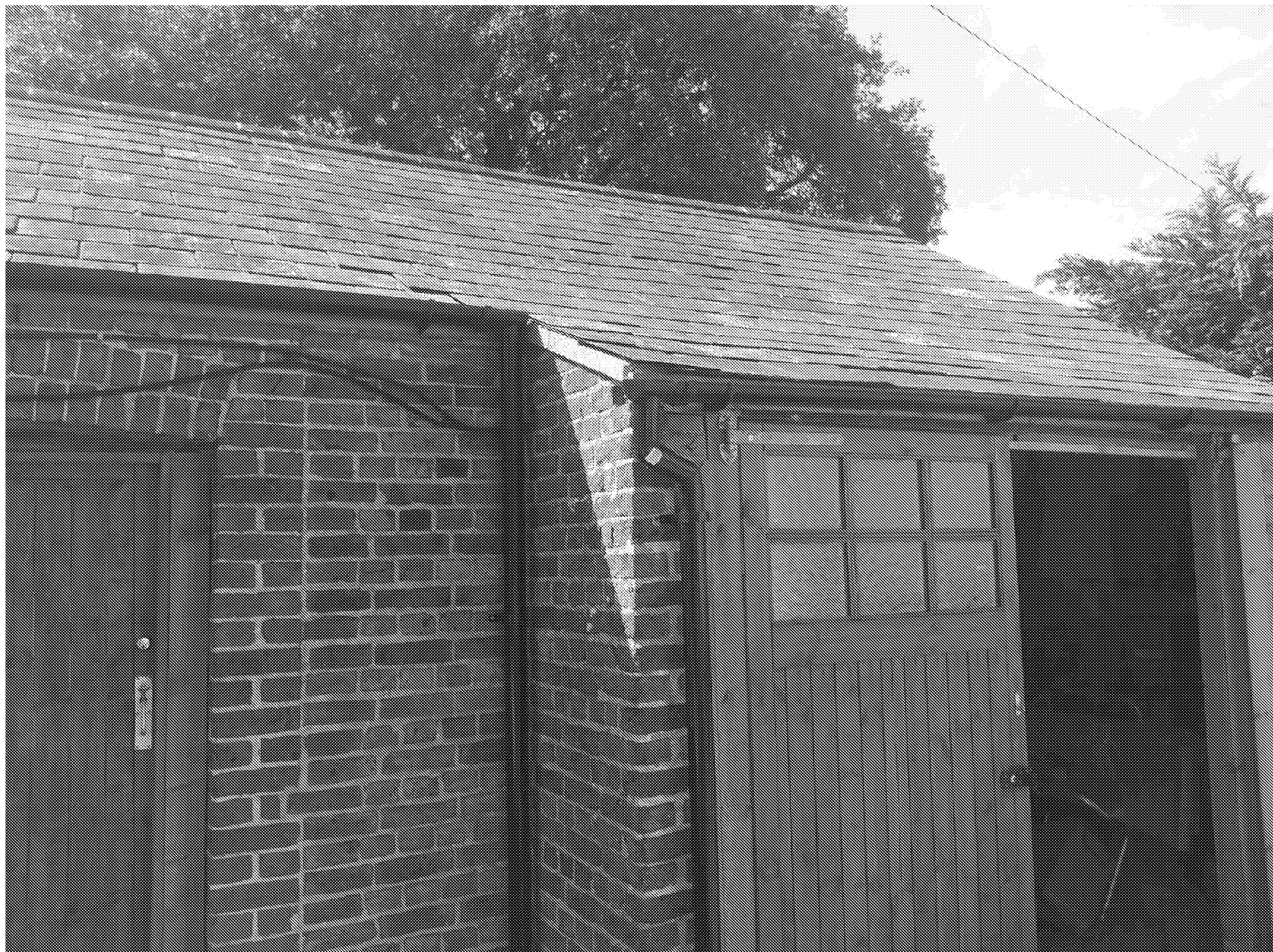
External view of Building 1
