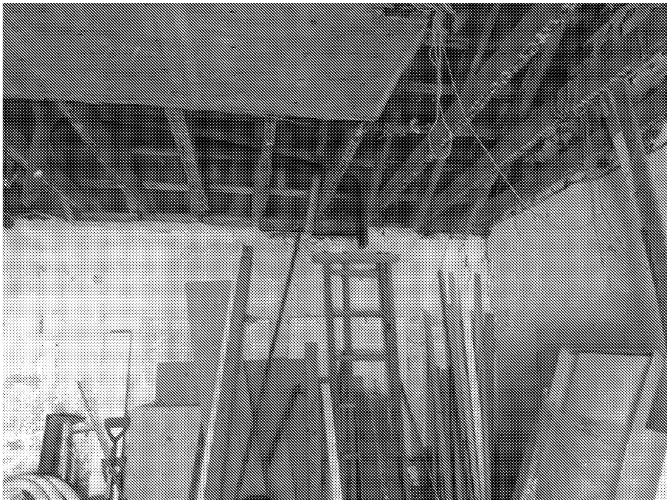
Internal view of Building 1
