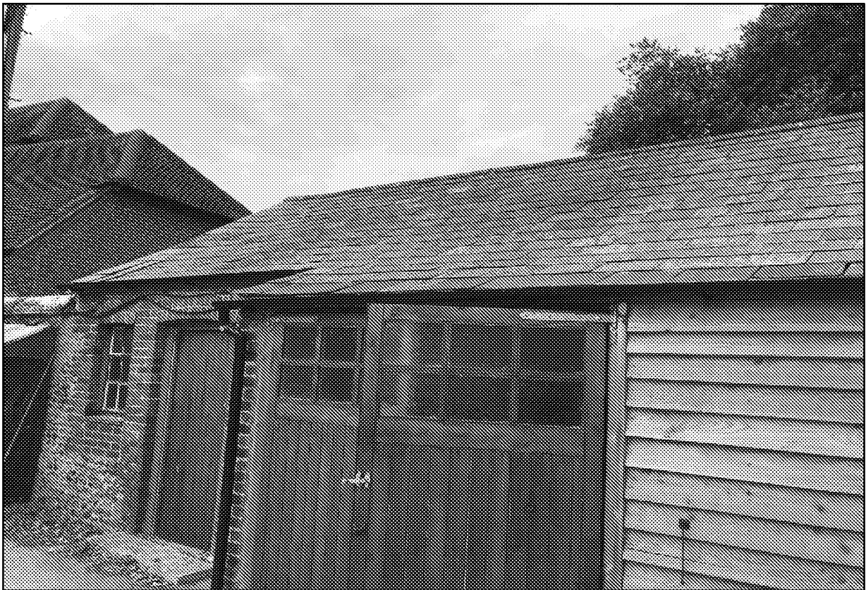
Photograph 8. The east roof face of Building E. Note the tight weatherboarding on the right of the photograph.
