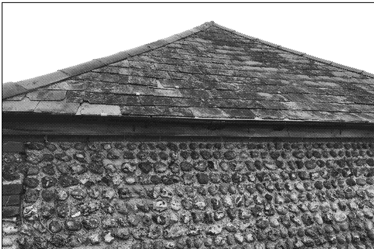
Photograph 5. The north roof face of Building D.
