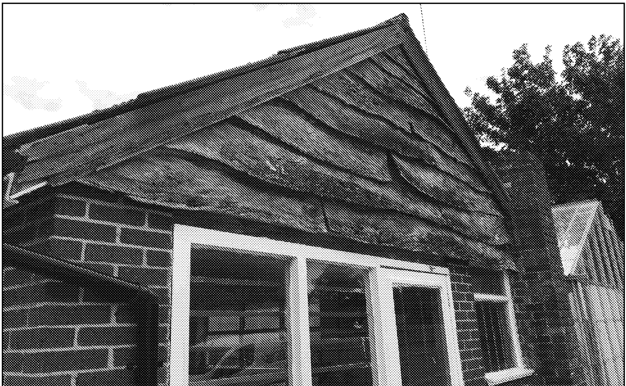
Photograph 2. The weatherboarding on the west gable of Building C.
