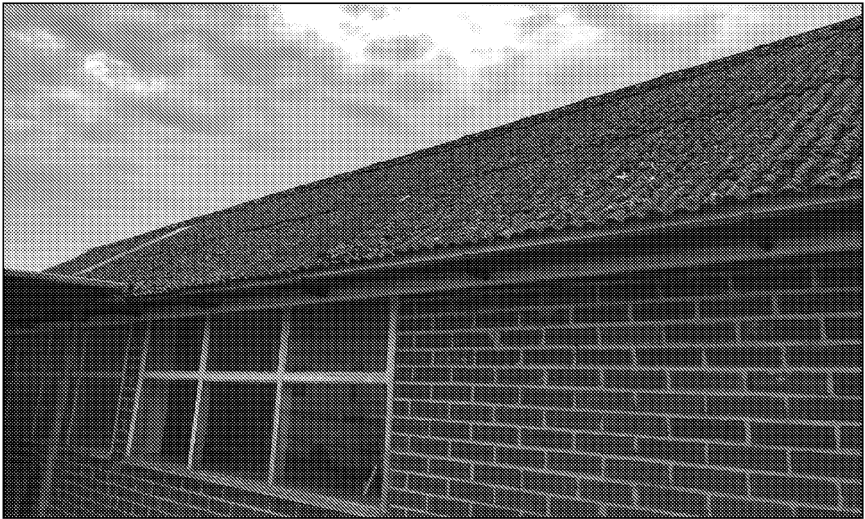
Photograph 1. The north elevation of building C showing the pitched asbestos roof.
