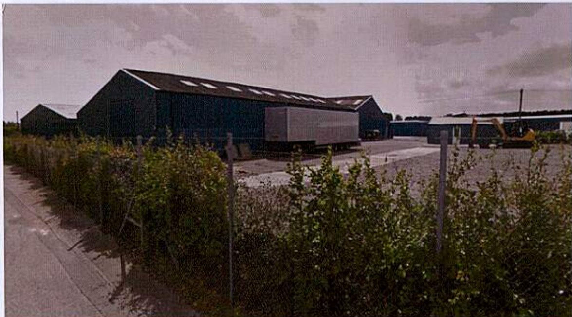
Fig 3. Looking across the site to the existing Clubhouse building unit 35 from Lillian Terrace. The new unit 35a has since been completed.
