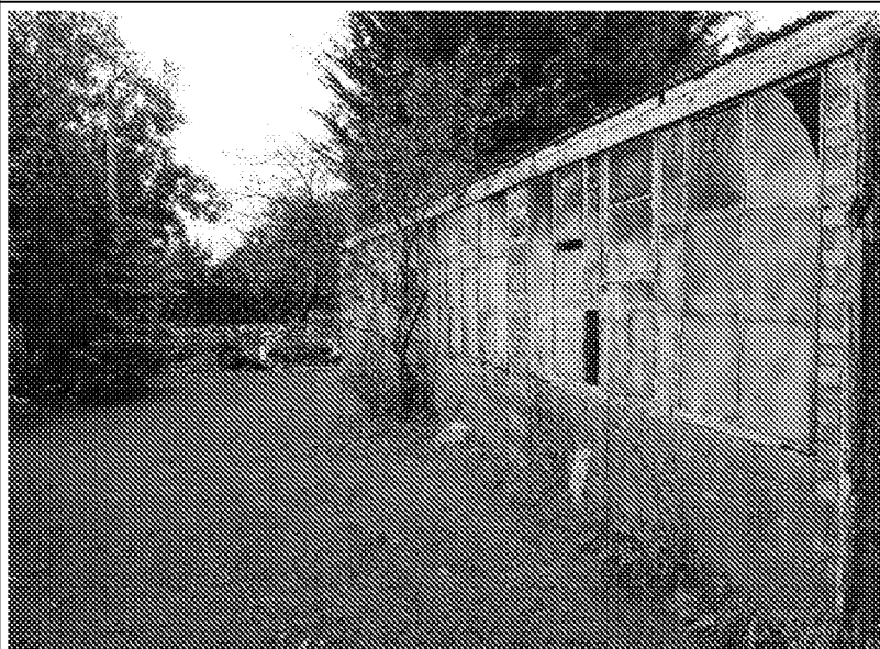
Former nursery building in western part of site
