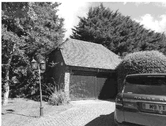
Garage building - B3
