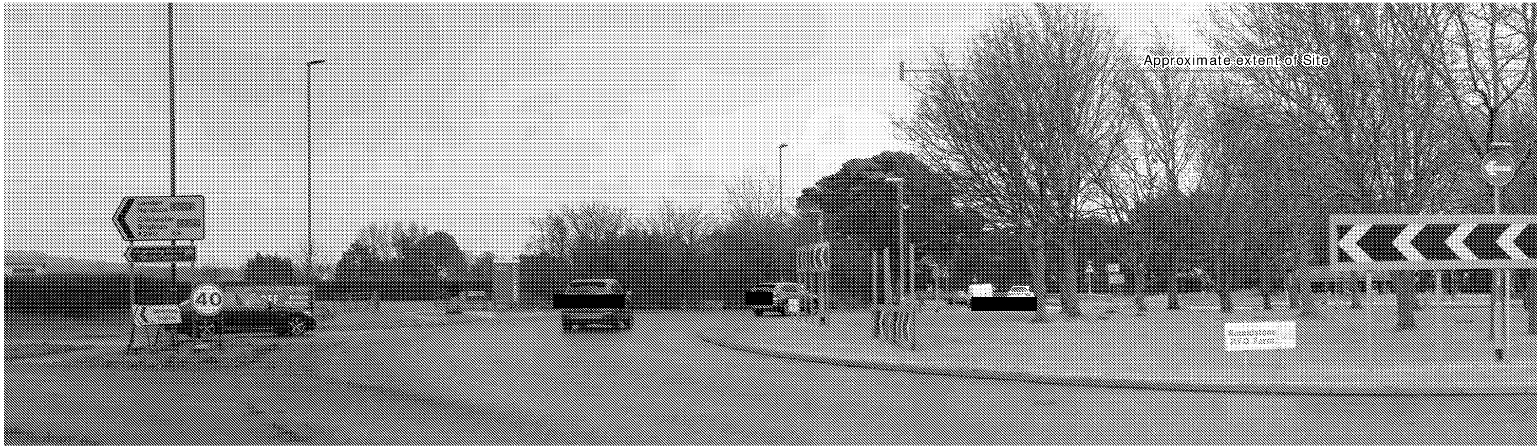
VIEWPOINT U1 Roundstone By-pass Road/A280 roundabout, looking southeast
