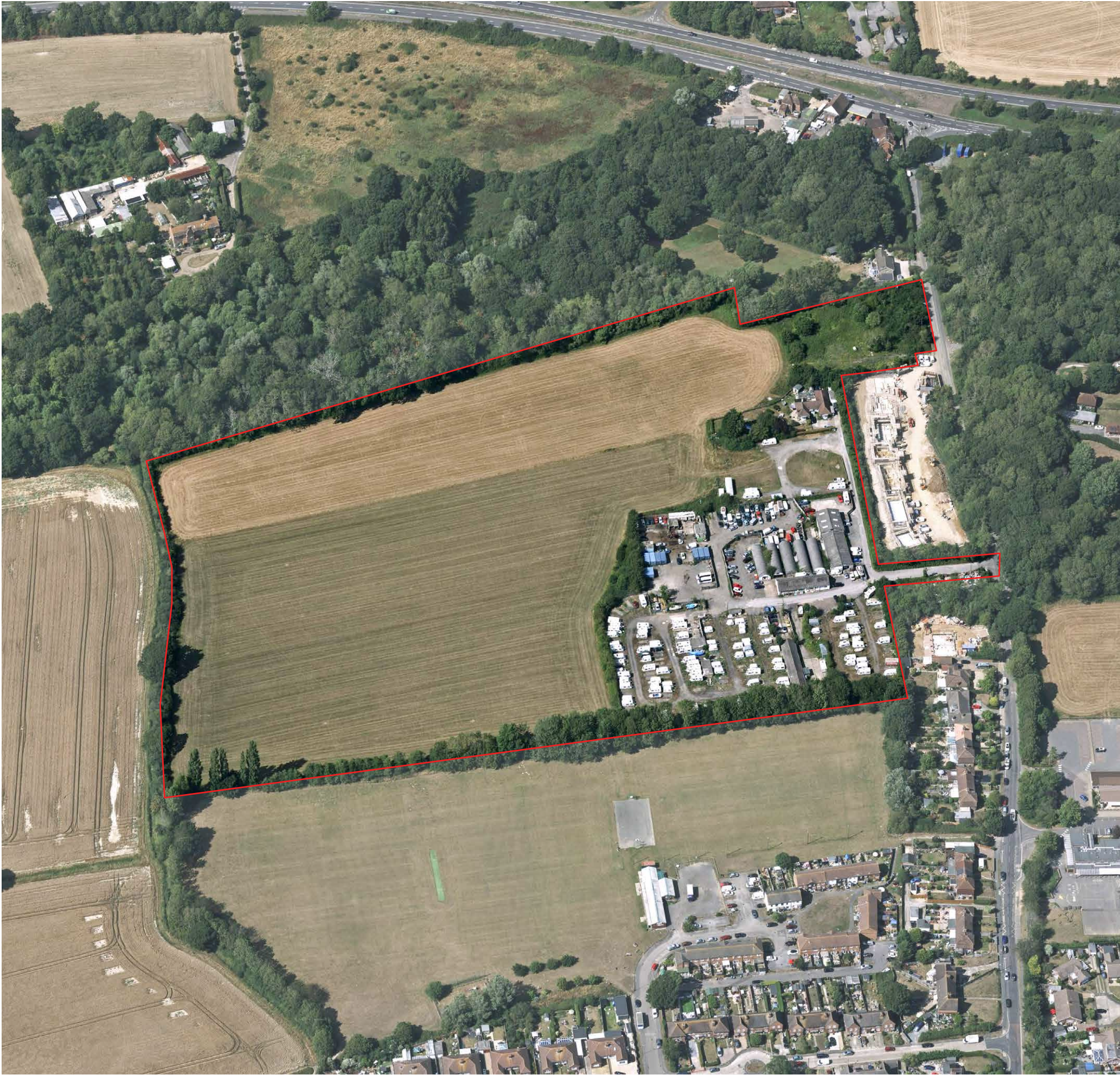
Aerial view of site and surroundings from the south
