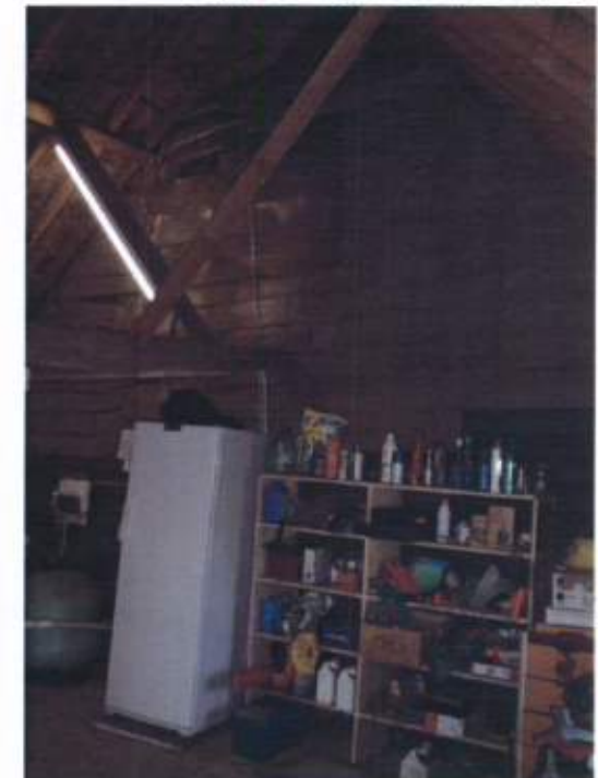
Fig.34: Timber clad adjoining wall of Workshop to Barn Note C.20th roof structure
