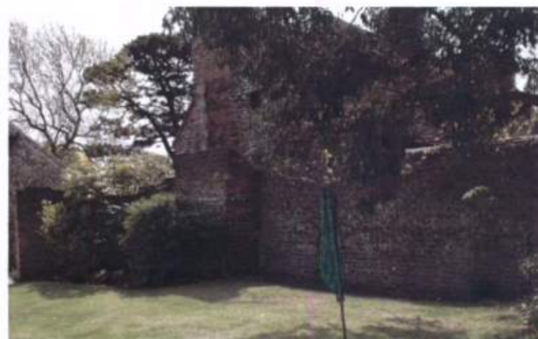
Fig.21: Garden wall from North showing anomalous returns now forming an outdoor privy
