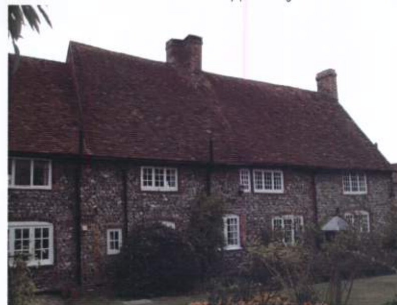
Fig. 13: Rear (West) Elevation; note straight joint to r/h side
