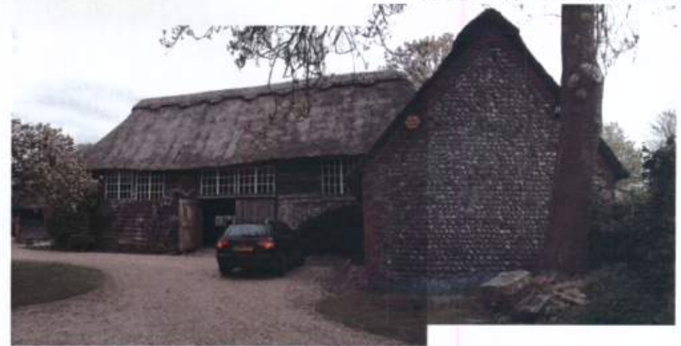
Fig.27: Barn flanked by Stable to the right and workshop to the left as viewed from entrance drive
