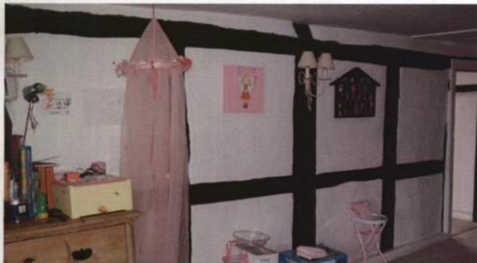
Fig.7: Former external wall at first floor
