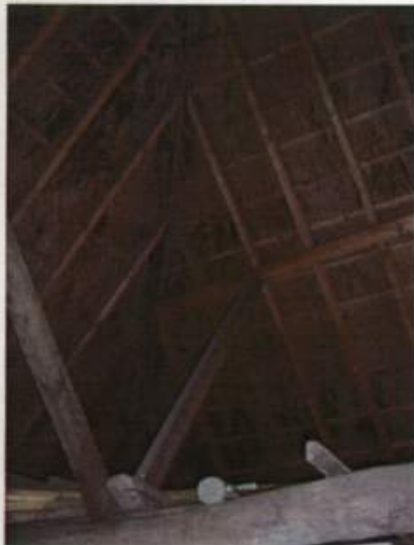
Fig. 17: Modern roof structure to Workshop
