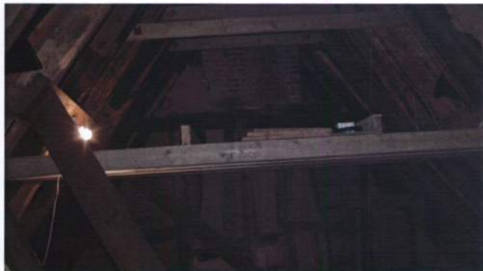
Fig.8: Remnants of former smoke bay to back of stack
