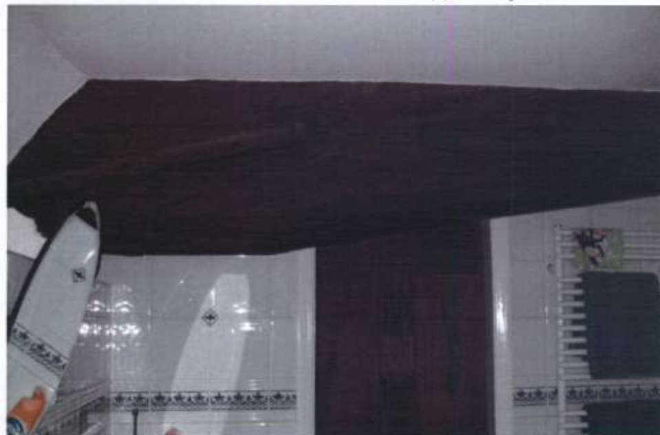
Fig.6: Base of tie beam to West side of house
