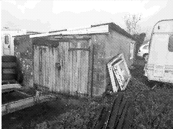
Photo 30: Building B7 looking north.
