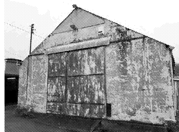
Photo 12: Western elevation of Building B3.
