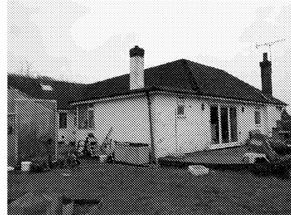
Photo 20: Northern and western elevations of Building B1.
