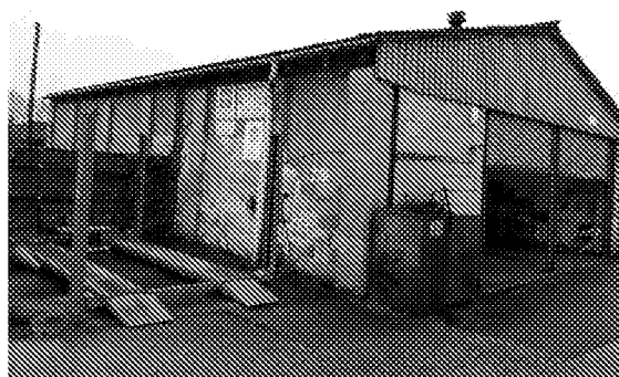
Photo 1: Southern and eastern elevations of Building B2.
