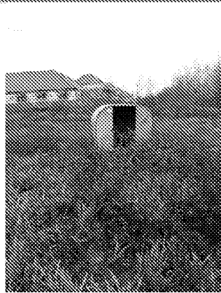
Photo 67: Building B14 looking east.
