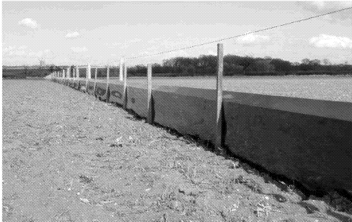
Figure 7 – an example of the temporary fencing material that will be used.
