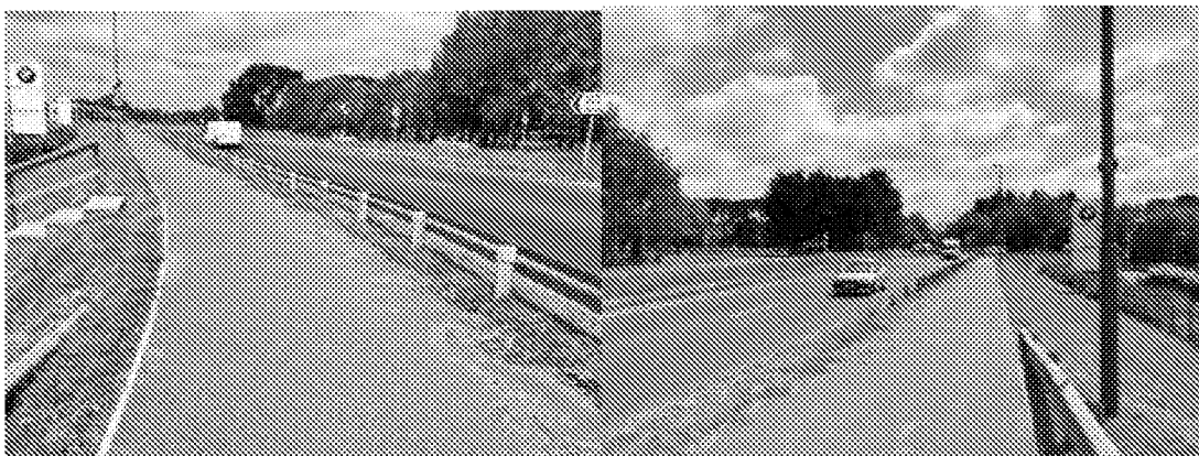
View of proposed location of southern side of toucan crossing, with gap in vehicle restraint and also steps to retail park
