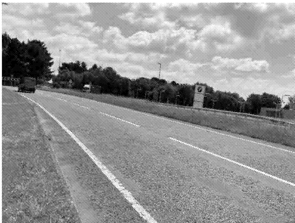
View of location of proposed toucan crossing facing east (west of Mill Lane Roundabout)
