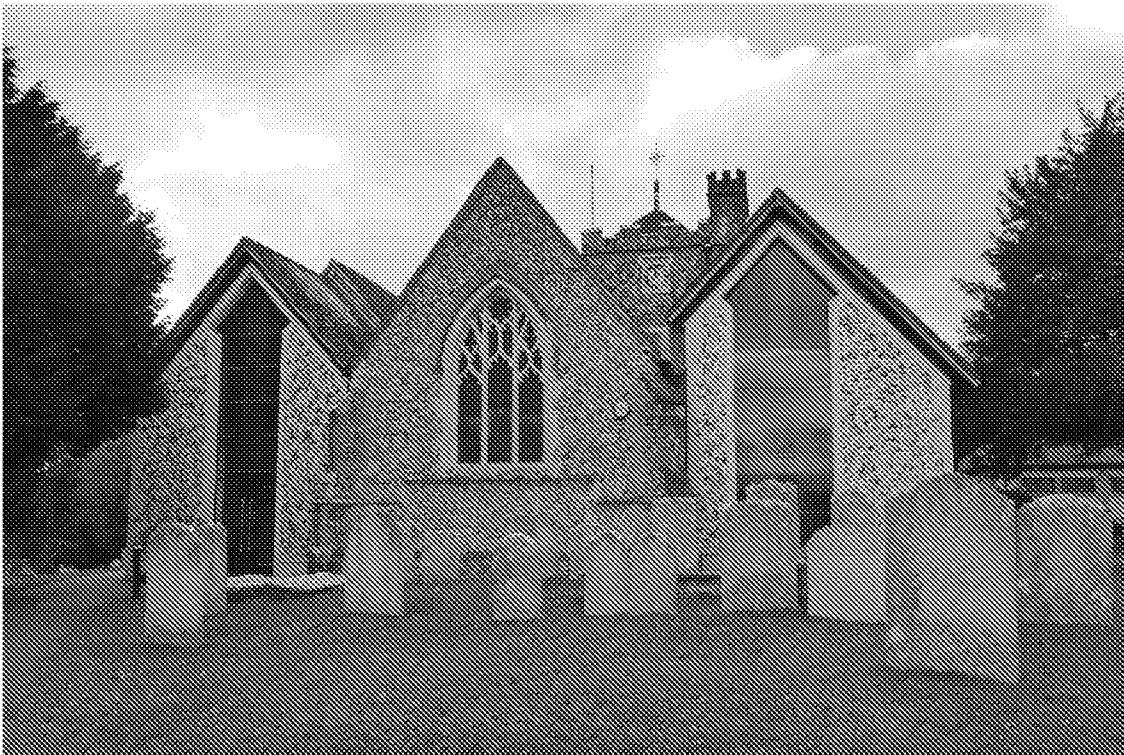
Figure 20: Grade II* listed church of St Margaret with modern extensions
