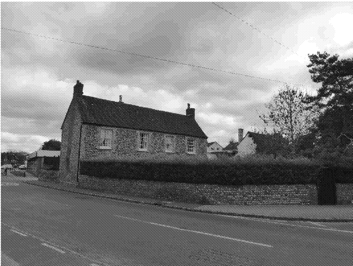
Figure 35: Grade II listed Eachways and front boundary wall from Water Lane looking south-east
