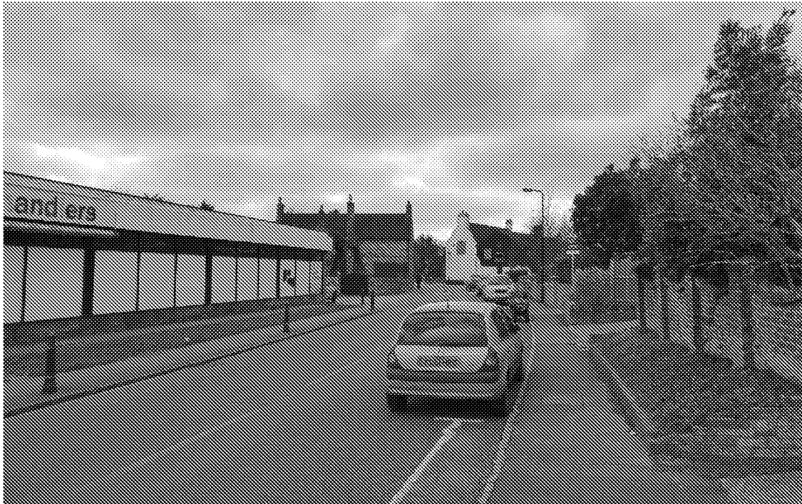
Figure 13: 'Gateway' to the Angmering Conservation Area from Water Lane
