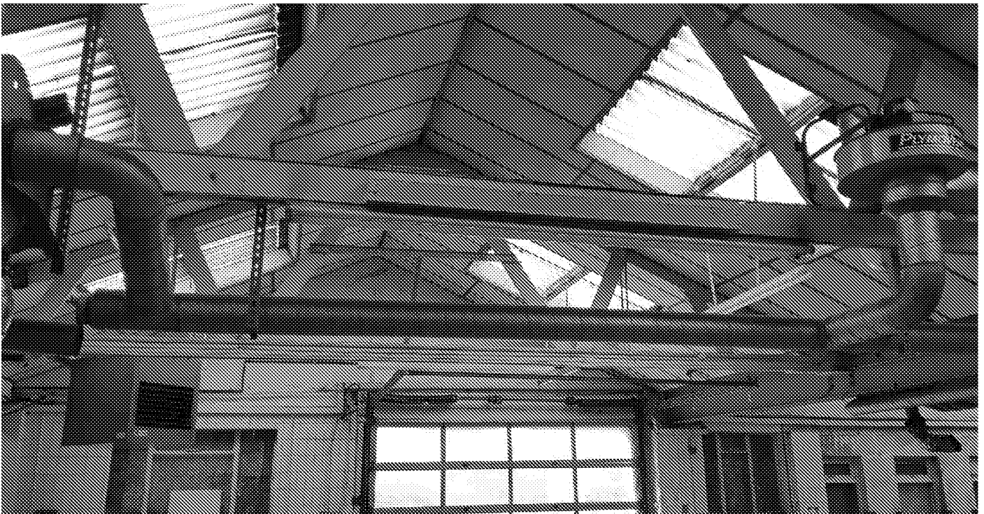
Photograph No. 2 - View of B1 ground floor roofing with no potential areas suitable for bats.
