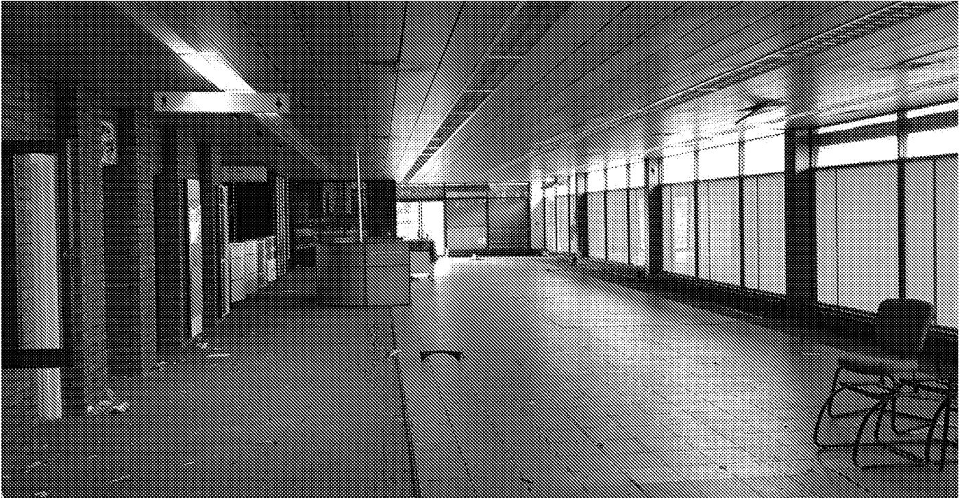
Photograph No. 1 - View of B1 first floor roofing with no potential areas suitable for bats.
