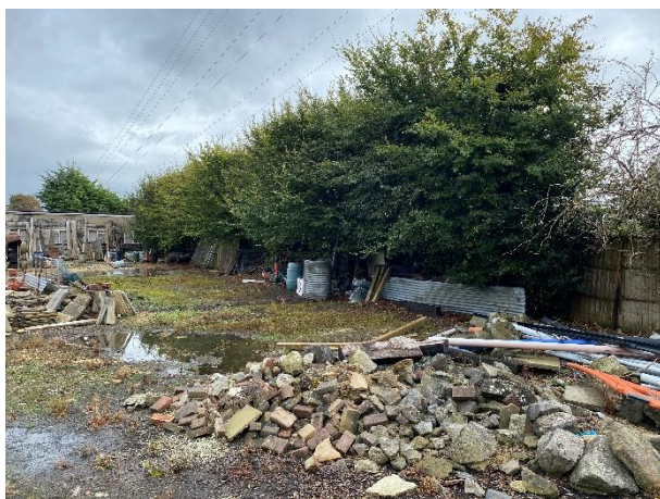
Photo 1: Example pile of rubble (Tn1, 4 and 5)
