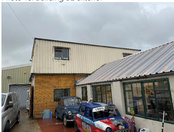
Photo 17: Building B5 exterior
