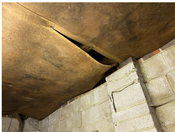
Photo 14: Building B1 interior
