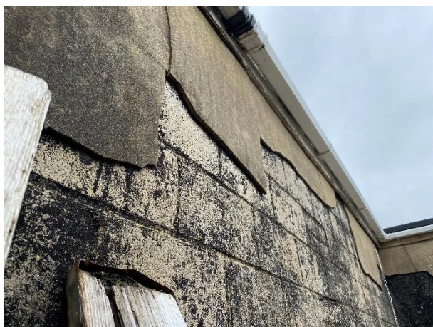
Photo 13: Building B1 exterior
