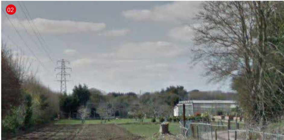
2. View showing the existing structures on site.
