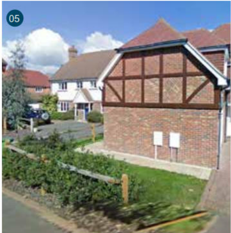
5. Brown brick with timber detailing
