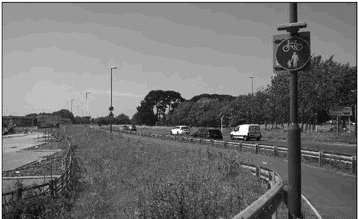
Figure 3.1: Shared Footway/Cycleway adjacent the A259 New Road
