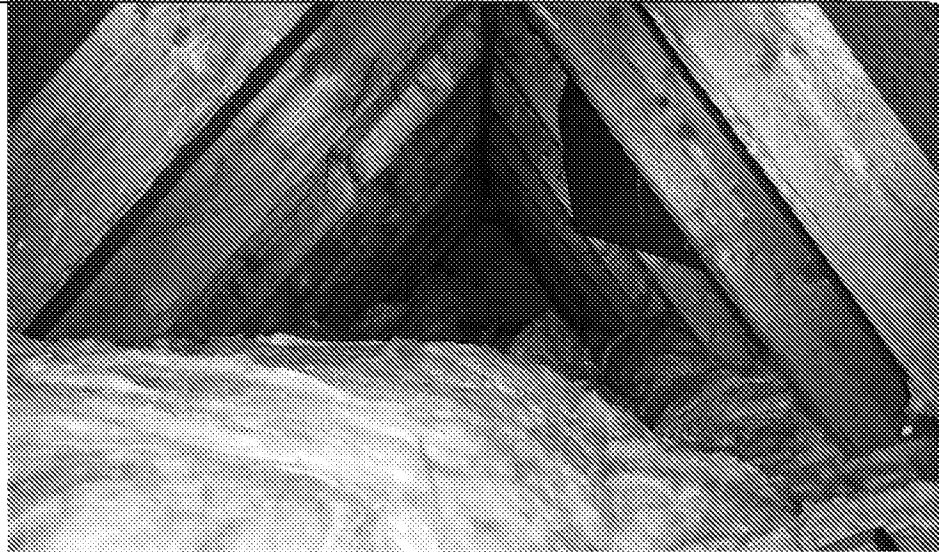
Photograph 6: Another section of the roof void with no evidence of bats.
