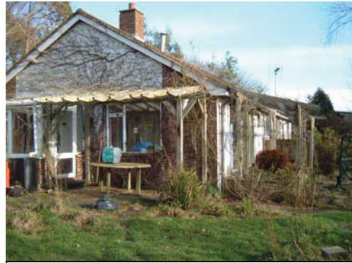
Existing Bungalow – (North/West - Side view 1)
