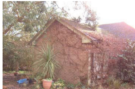
Existing Bungalow – (North/East - Front view 2)
