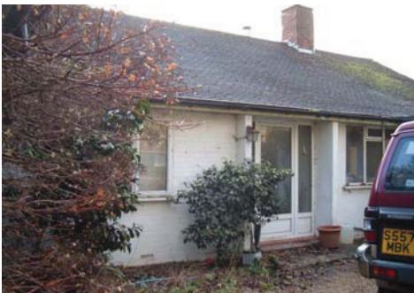
Existing Bungalow – (North/East - Front view 1)
