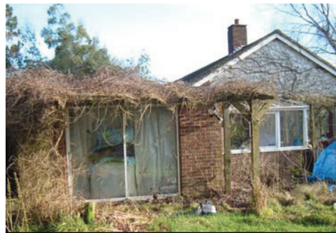
Existing Bungalow – (North/West - Side view 3)
