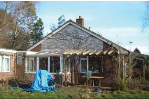
Existing Bungalow – (North/West - Side view 2)
