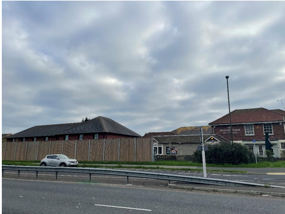
Looking south from the A259 towards the northern elevations of the main hotel and restaurant
