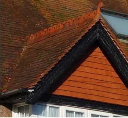
Dark coloured bargeboard
