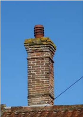
Chimneys on key plots
