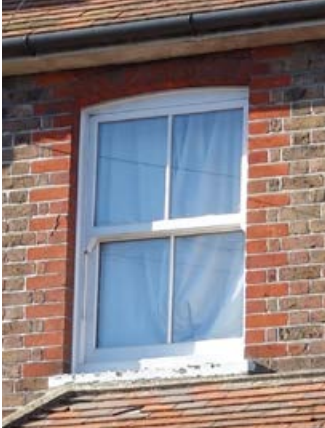
Brick detail window surrounds
