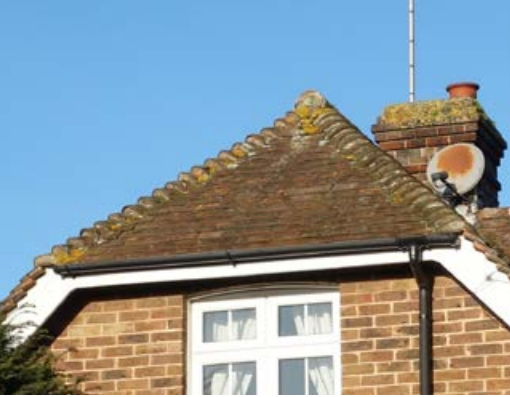
Barn hipped roof
