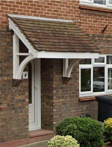
Lean-to pitched porch canopy
