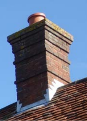
Chimneys on key plots
