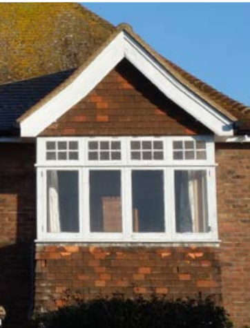
Pitched roof to gabled bay windows
