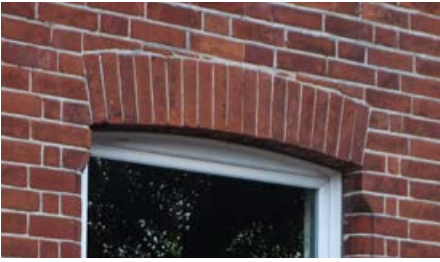
Gauged brick arches
