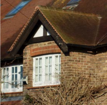
Pitched roofs to gabled bays
