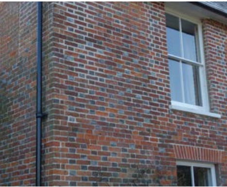
Red brick building with blue header 'diaper' pattern
