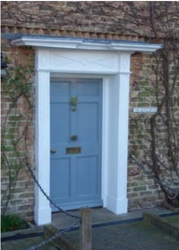
Generally flat roof porch to front door
