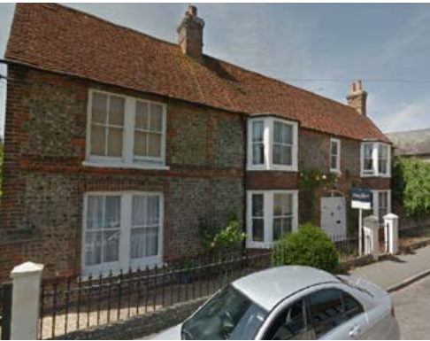
Flint building with brick quoins
