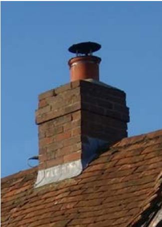
Chimneys on key plots
