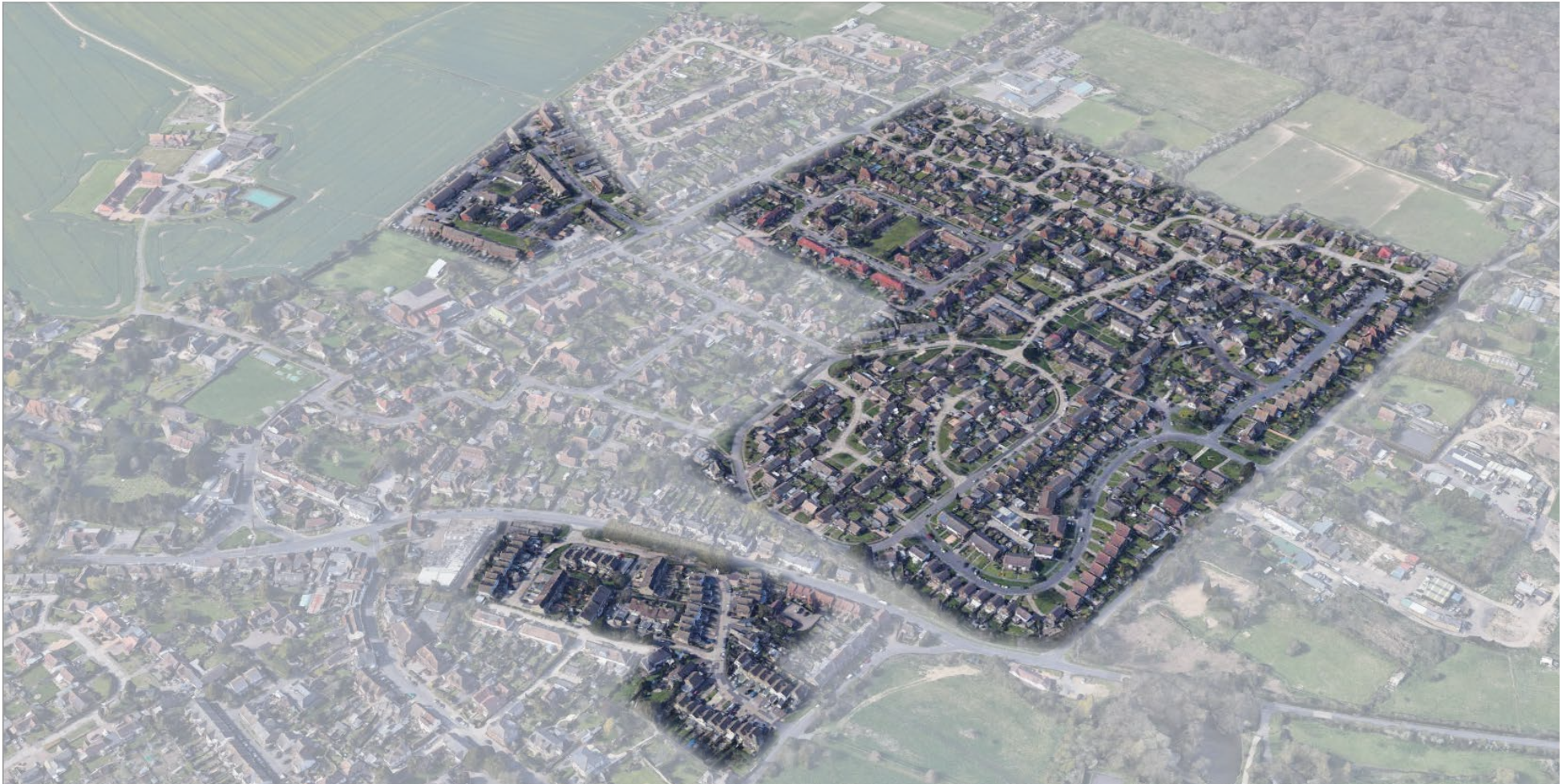
Aerial view (Google Earth)
