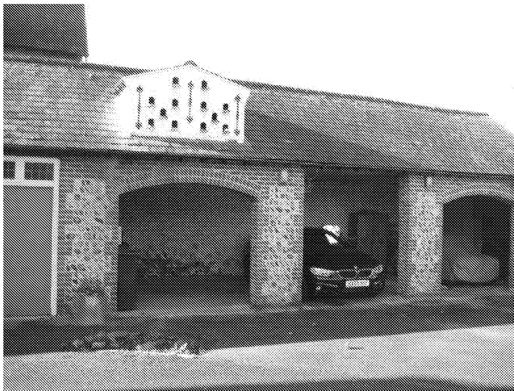
Photograph B4 – Garage / Carport – East Elevation
