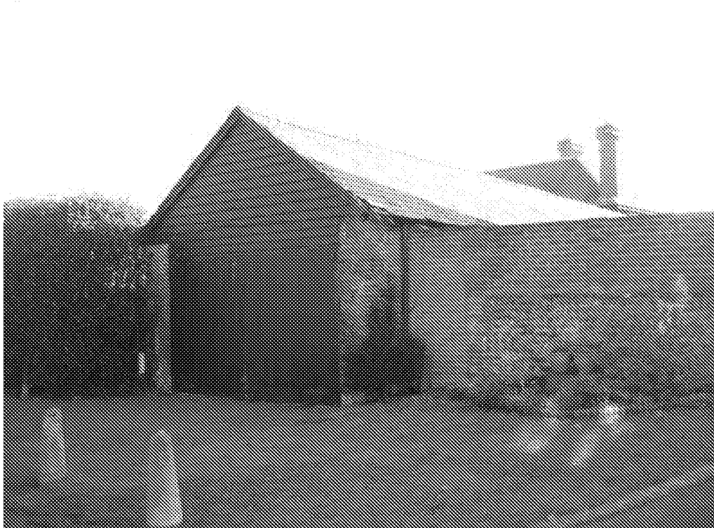
Photograph B6 – Garage / Carport – North Elevation
