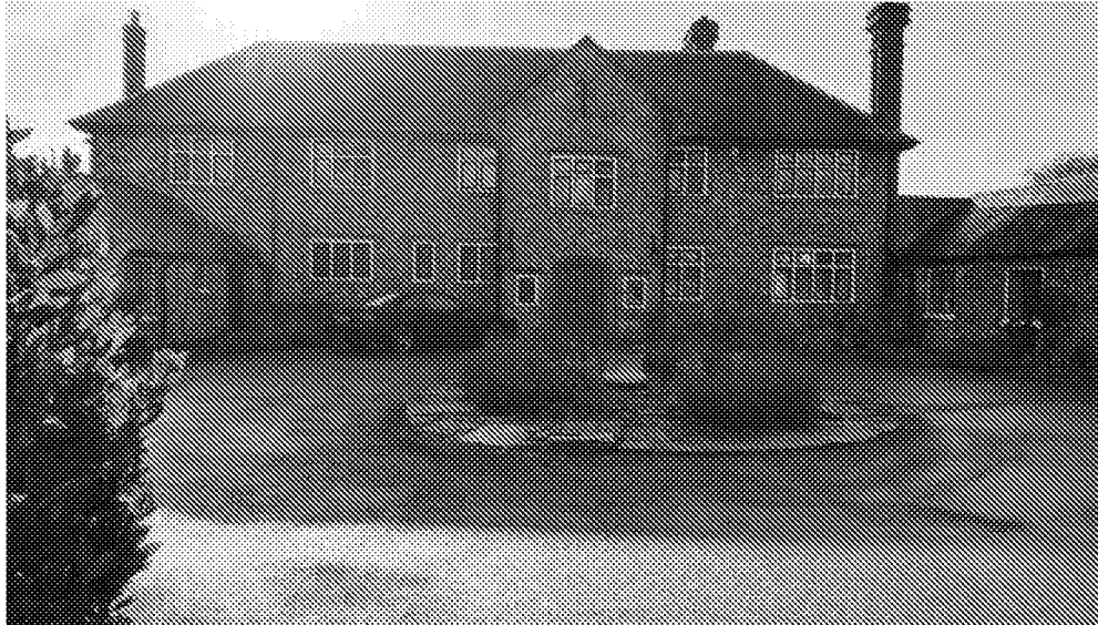
Photograph B1 – House – Front (North) Elevation
